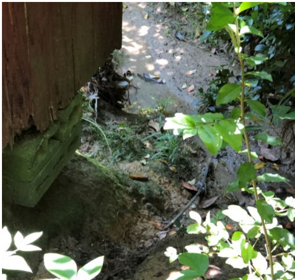
Figure 3. Photograph of back yard shed where foundation block is experiencing erosion from the stormwater ditch.
