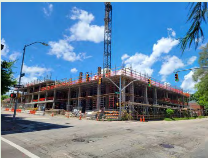
The Hilton Garden Inn / Homewood Suites under construction on McDowell and Davie streets
