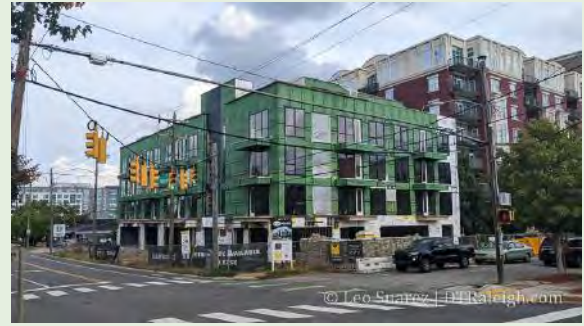
615 Peace under construction Photo by Leo Suarez
