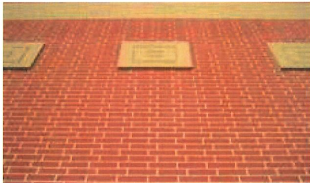
A raking stretcher bond appearance with finished foam shapes to accentuate the wall
