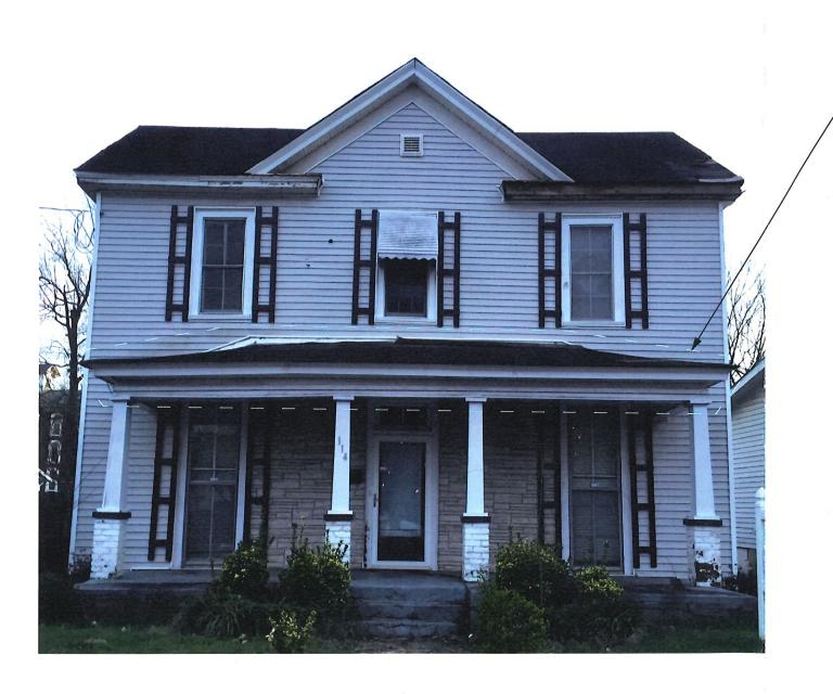
PORCH ROOF MUST BE REMOVED FOR HOUSE MOVE. TO BE RECONSTRUCTED AT TIME OF RENOVATION TO MATCH EXISTING PORCH ROOF DIMENSIONS AND MATERIALS.
