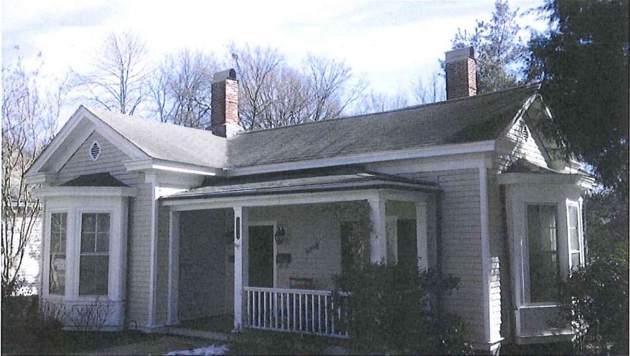
Photos of existing conditions:
