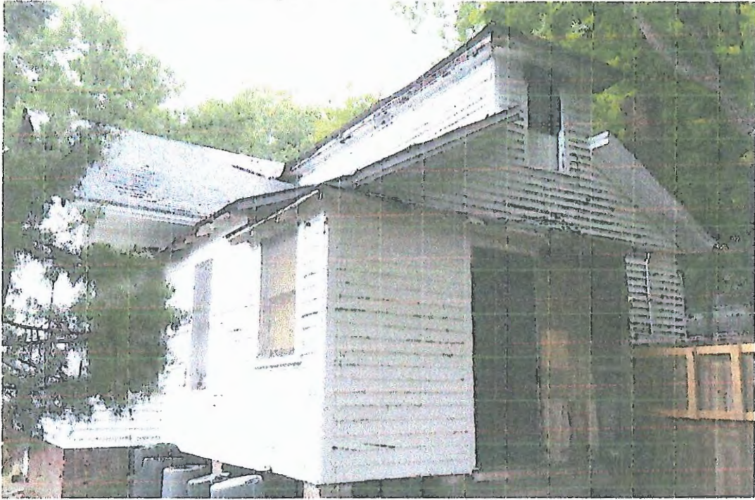
South Elevation, back of house an SW Corner
