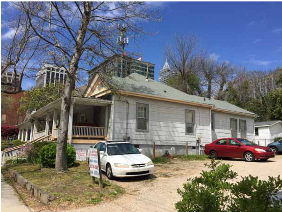
219 E Cabarrus - Seen where rear gable is held below the main cross gable
