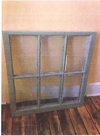
Figure 7: New window sash
