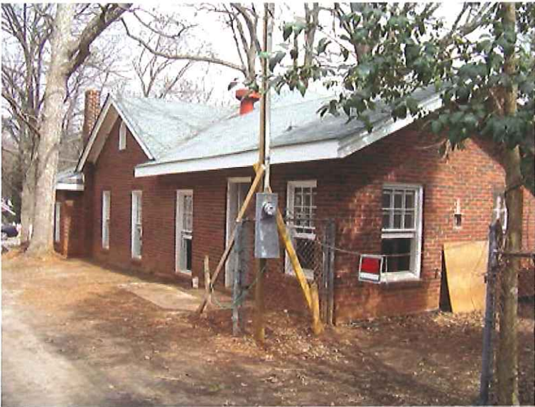
West and partial south elevation
