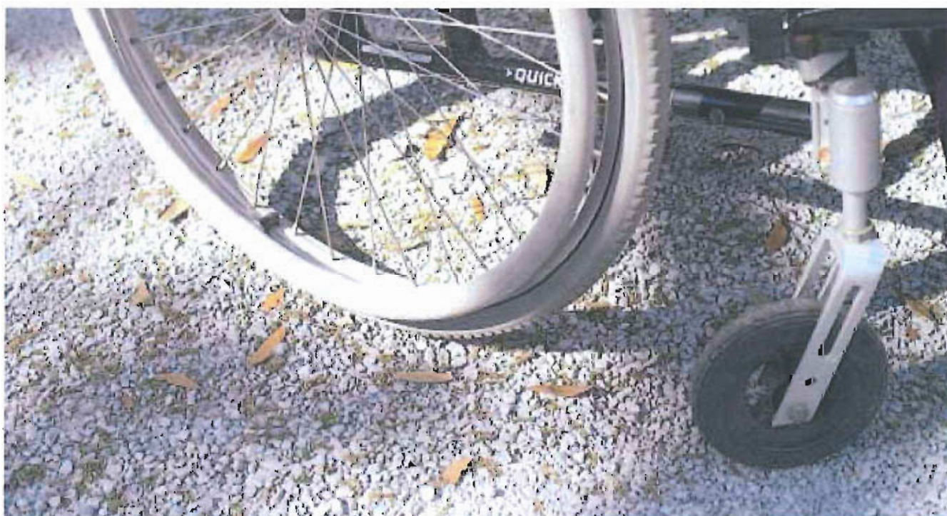
Wallace Residence, Savannah, GA—Gravelpave 2 creates a wheelchair-accessible surface by stabilizing gravel and supporting tire pressure. 7% dry cement was mixed with gravel before filling rings. Cover photo: Westin Kierland Resort and Spa, Scottsdale, Arizona—Grasspave 2 tire lane and Gravelpave 2 tire lane (concrete widening).
