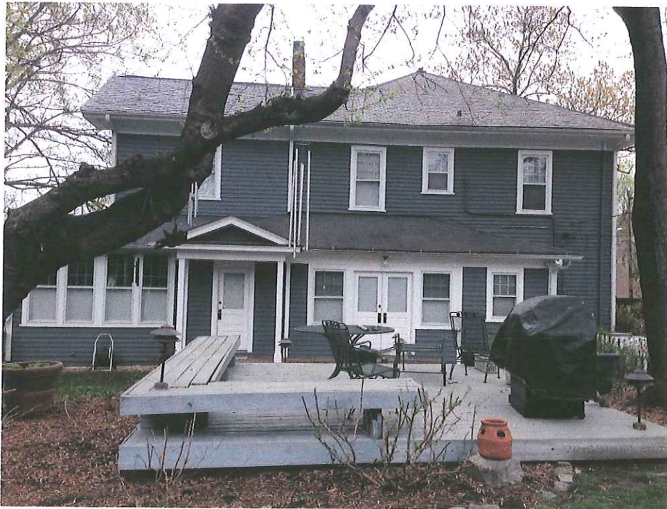
The bottom right window on the rear facade of 525 N. Bloodworth is the focus of our project. This double-hung window will become a fixed window. All trim, siding, and paint colors will remain the same or match existing in all material properties.
