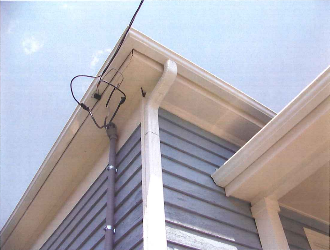
Existing trim at front corner of residence, original crown molding
