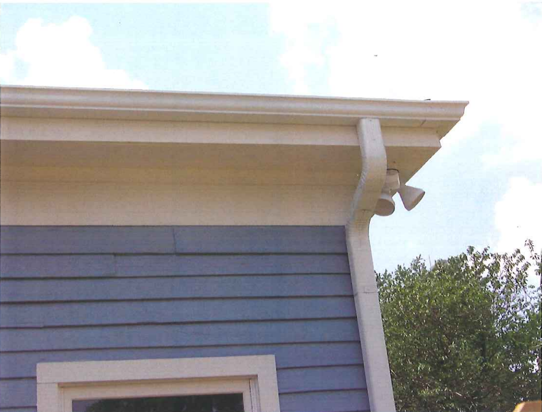
New flat band trim at new addition at rear of residence
