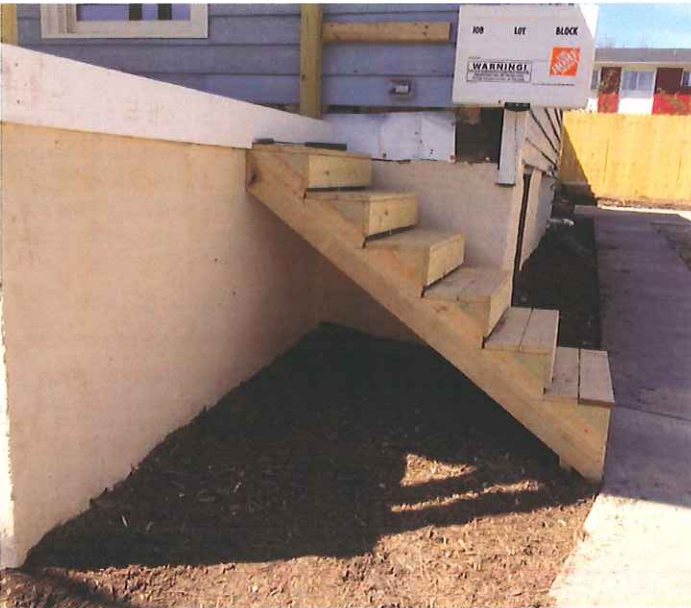
Straight run stair at driveway, removed
