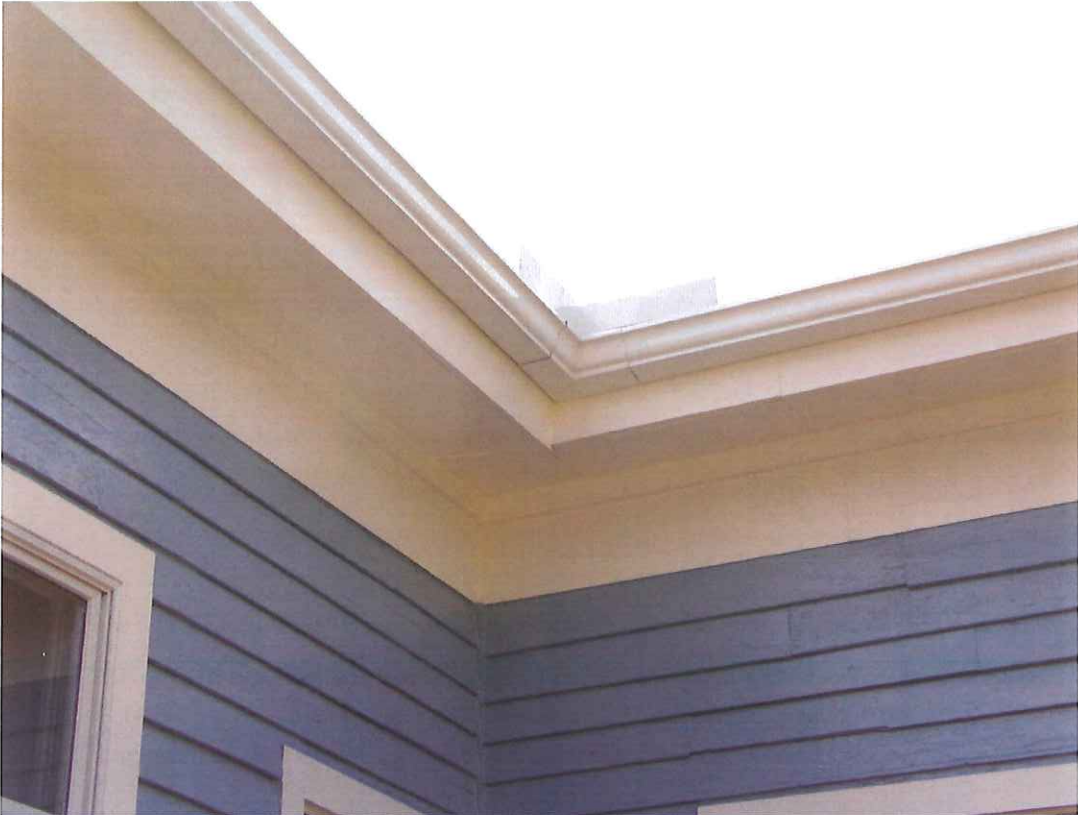
New flat band trim at new addition on rear of residence
