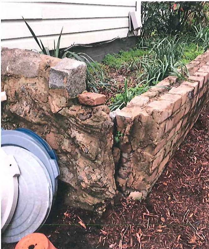
Figure 3: Existing 33-foot long wall to be demolished and replaced with new 12 feet long stone retaining wall.
