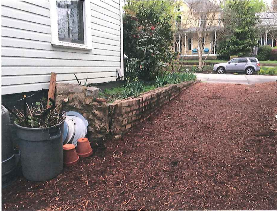
Figure 3: Existing 33-foot long wall to be demolished and replaced with new 12 feet long stone retaining wall.
