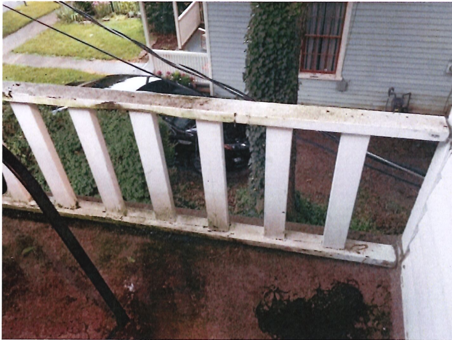
Height of balcony railing. 6" below IRC requirements
