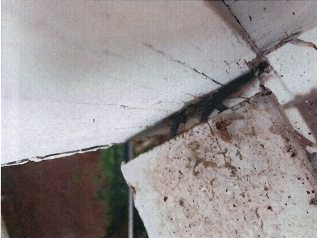
4 nails holding the balcony in place
