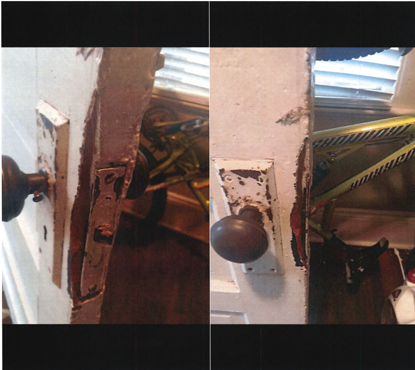
Front left door detail. Shows significant pieces missing from (what appears to be) forced open at some point.
