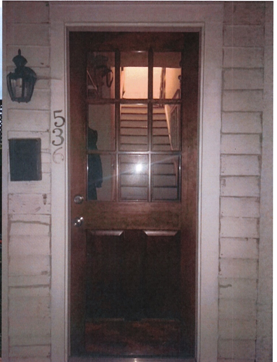
Replacement front right door – prior to painting of casing. Front right door after painting of casing. (Casing replaced in this instance due to deterioration.)
