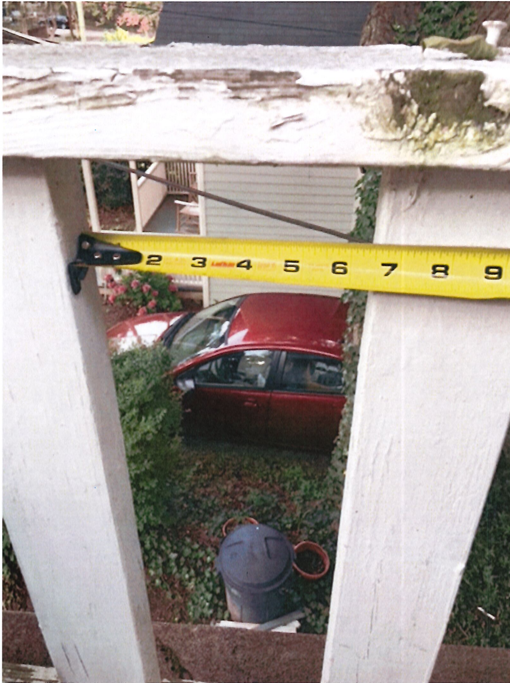
Width of space between balcony balusters.
