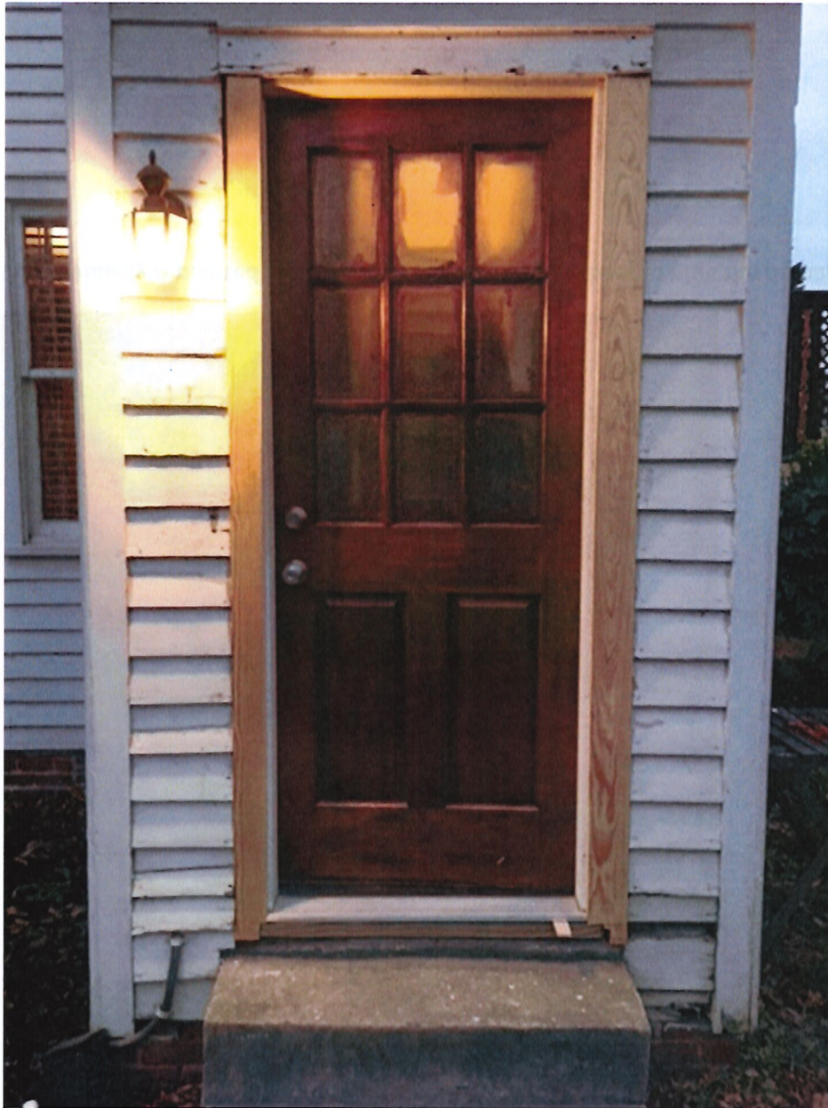
Replacement front right door – prior to painting of casing. Front right door after painting of casing. (Casing replaced in this instance due to deterioration.)
