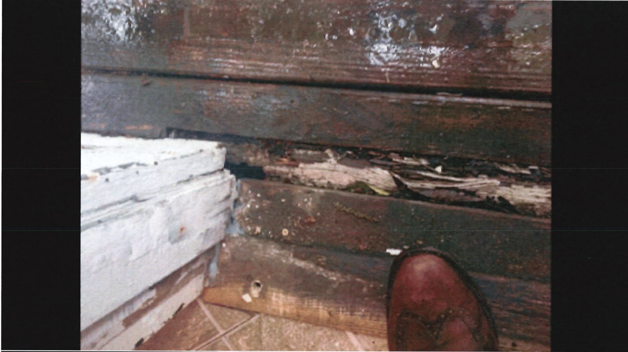
Rear door, and framing. Framing is representative of the deterioration of the bottom of the door. Both were soft to the touch
