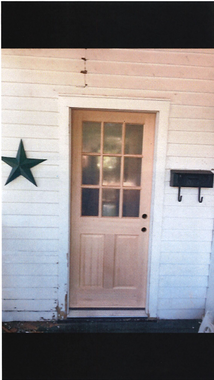
Front left door prior to staining (notice reuse of the casing.
