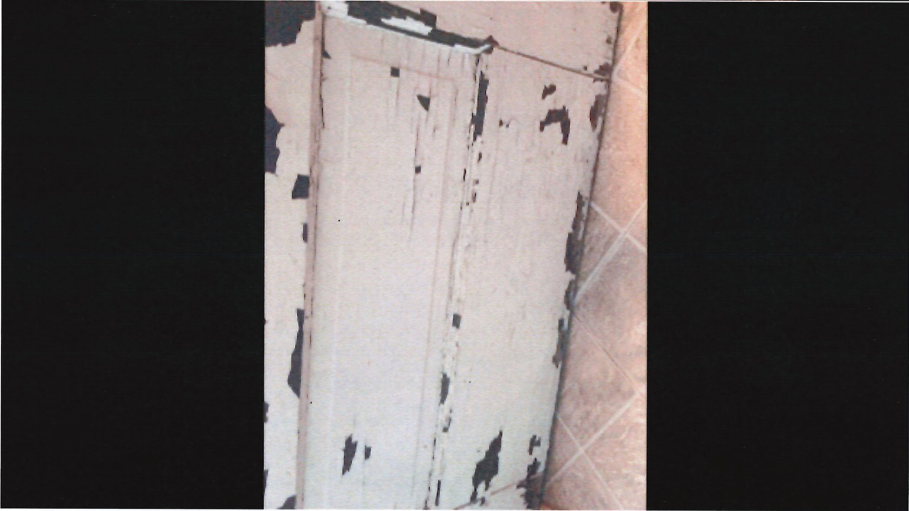
Rear door, and framing. Framing is representative of the deterioration of the bottom of the door. Both were soft to the touch
