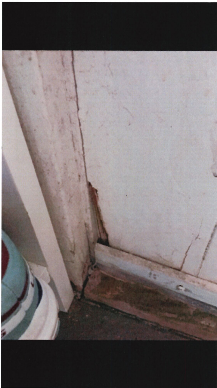
Large chunk missing from inside front right door. Also shows more cracking and extra wooden bracing applied to help keep the door together.
