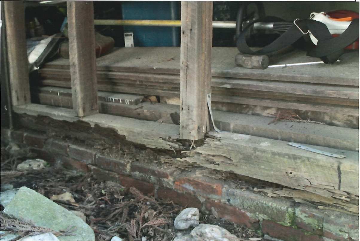
Deteriorated sill plate
