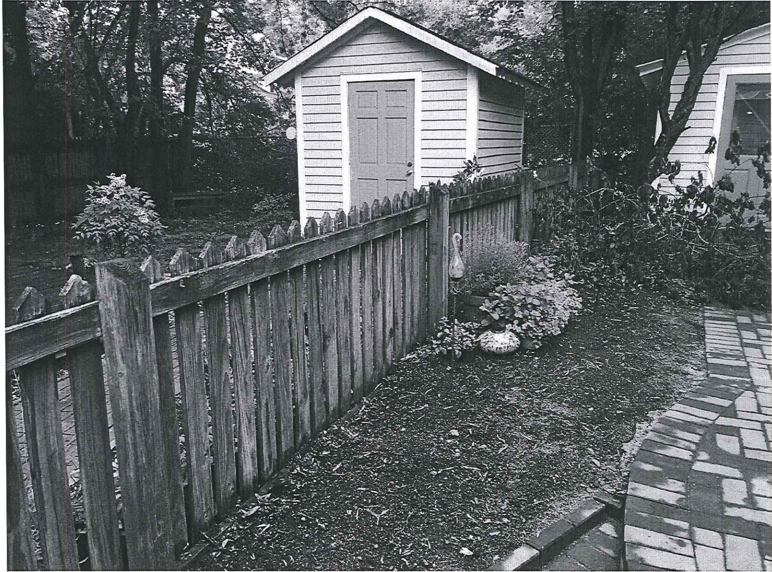
Existing Fence (Fig#1a)
