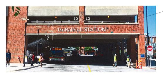
24" HIGH STAINLESS STEEL FABRICATED LETTERS WITH 1 1/2" RETURN - STUD MOUNT TO WALL
