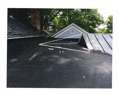
Existing conditions. Rotten wood on metal roof riser. Wet behind metal roof riser. Mold/mildew on metal roof riser.
