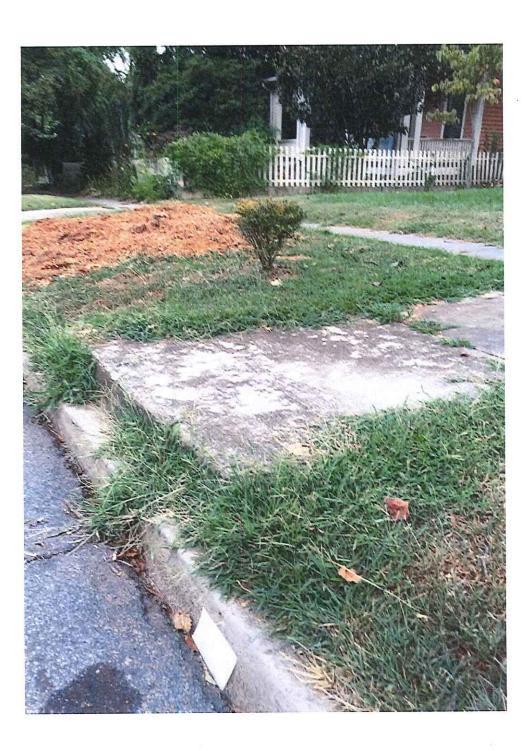
Driveway approach to be modified to flatten hump and reduce drag. Shape, texture and dimensions will be the same
