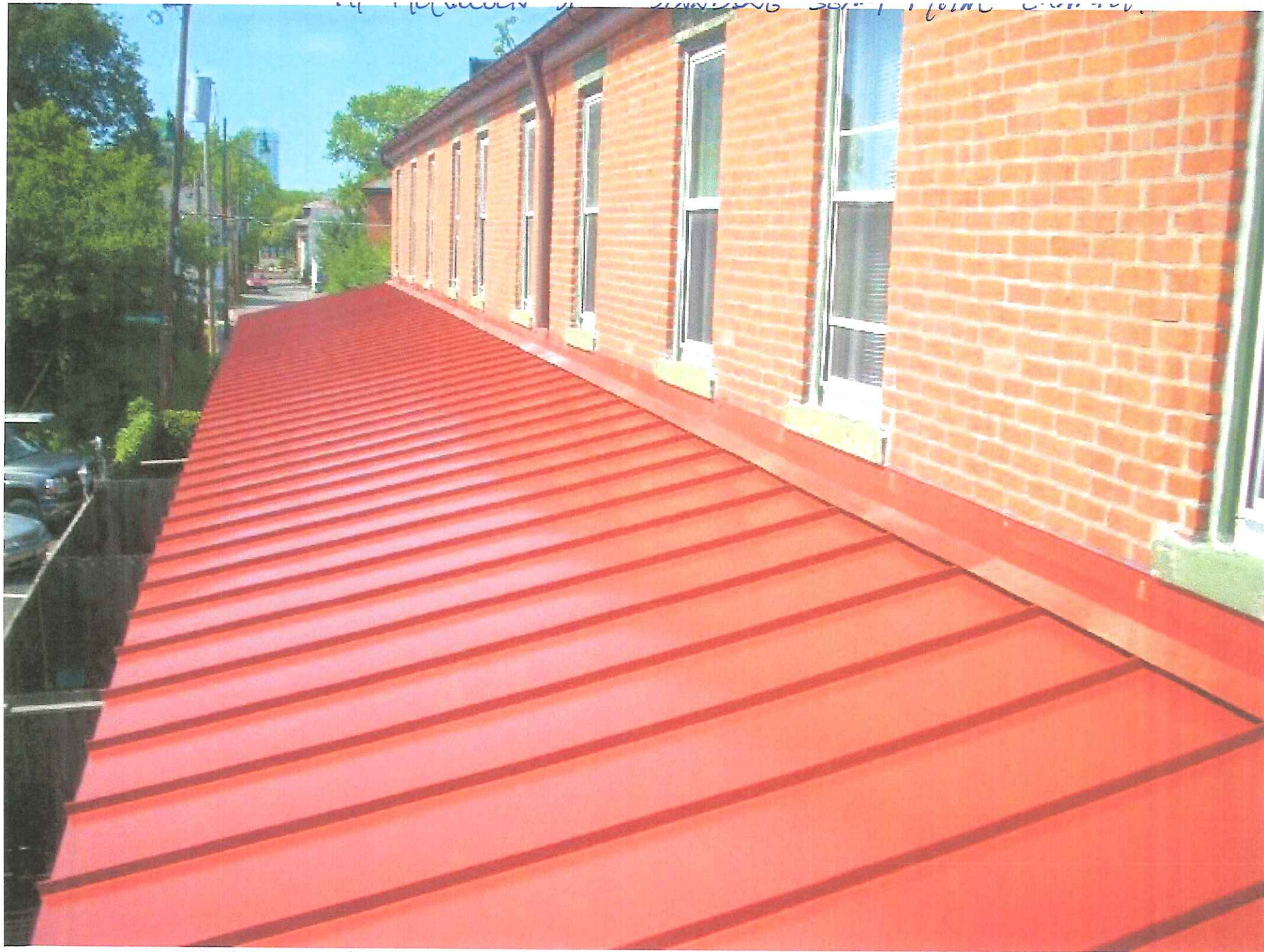
711 McCulloch St standing seam metal example
