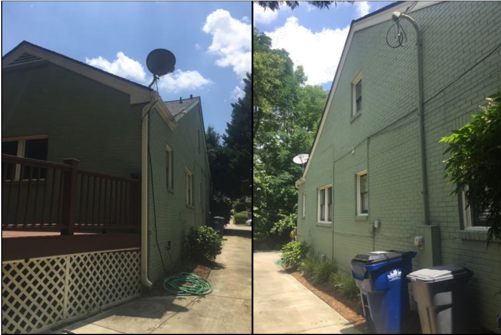
1 PHOTO-SIDE-DRIVEWAY (WEST) Scale: 1/32" = 1'-0"
