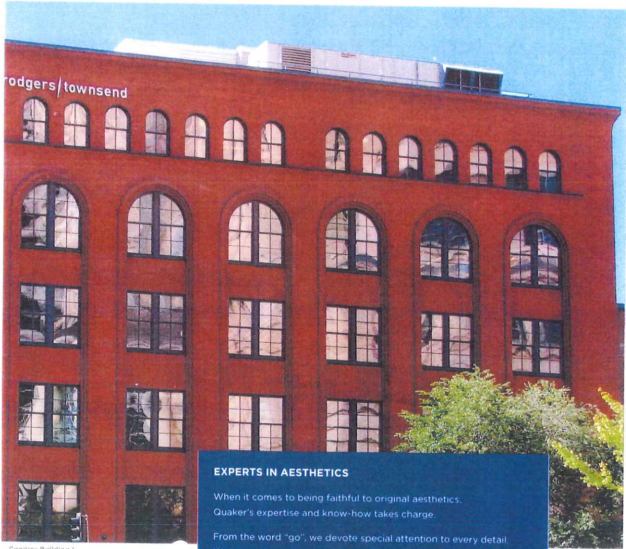
Cuppies Building 1 1101 Haynes Street Raleigh, NC 27601 100,000 sq. ft. / 1900s Historic Preservation / Adaptive Reuse
