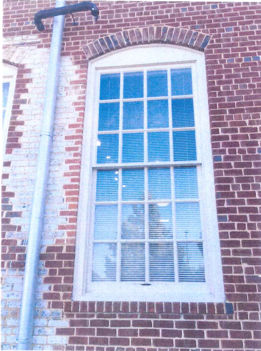
Exhibit 1: Existing window at Pilot Mill
