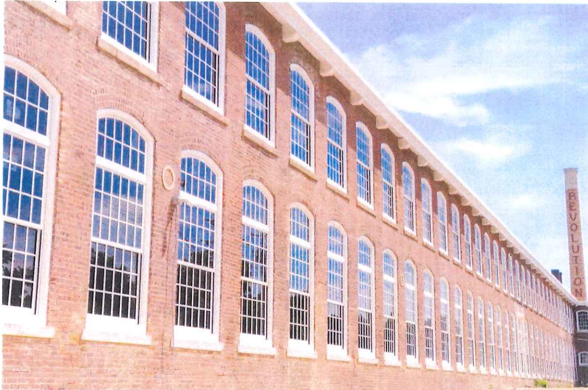
Exhibit 4: Revolution Mill, Greensboro, NC—NPS approved Quaker aluminum windows.
