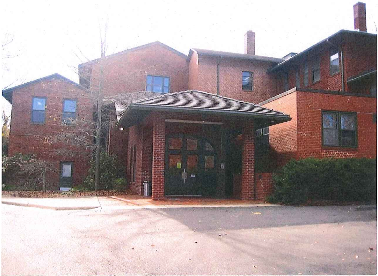
Front Entrance 1100 Bldg 2
