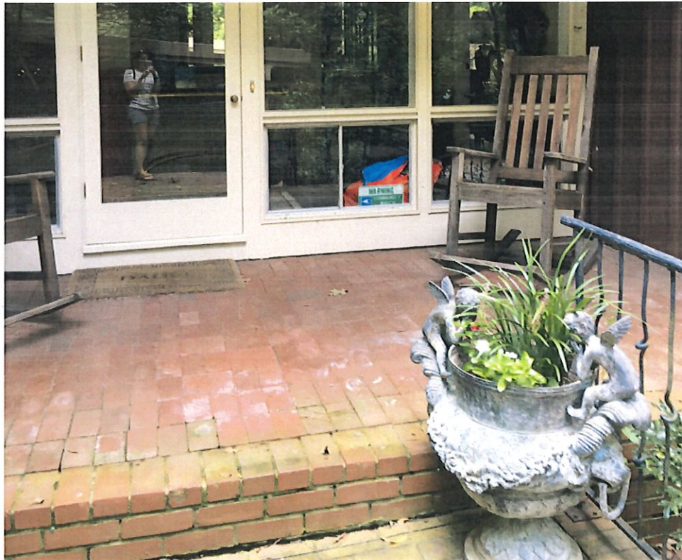
Raised walk separating from steps
