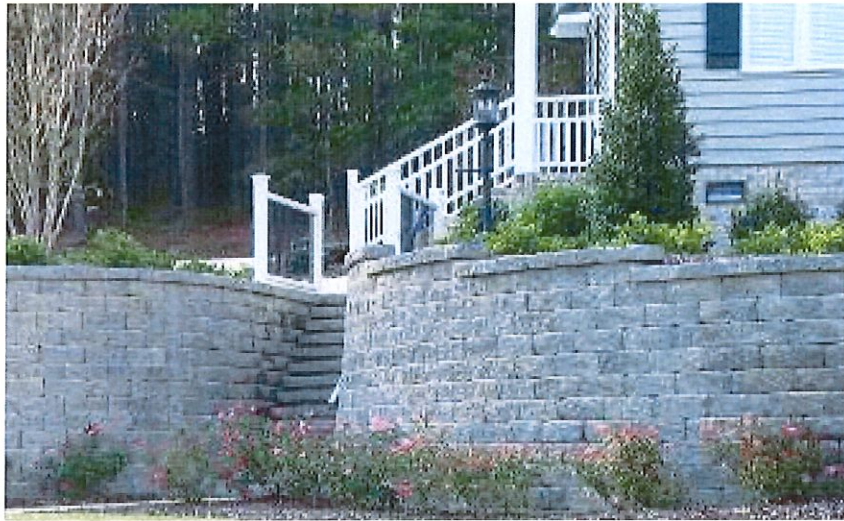
Versa-Lok, Standard in Colonial Color Block Dimensions: Width (face): 16" x Height: 6" x Depth: 12"
