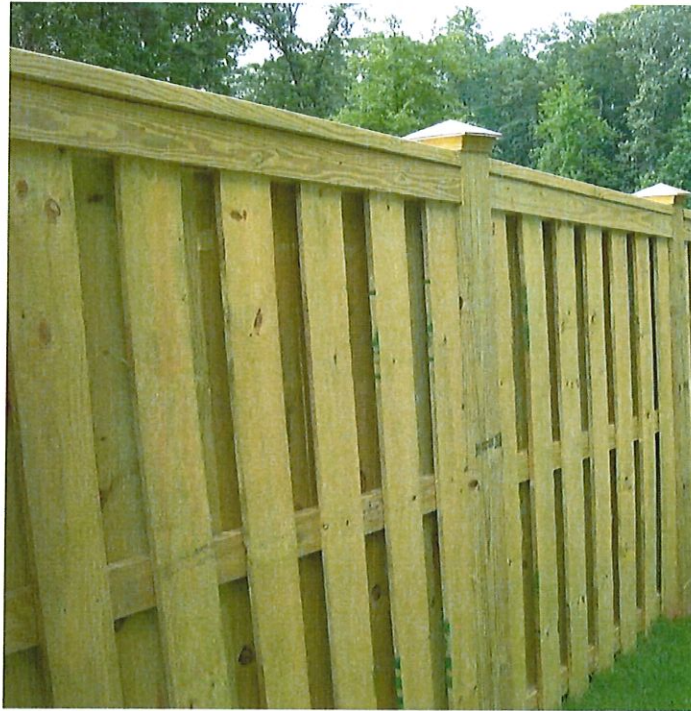
Privacy Fence – Example Constructed of pressure treated 6x6 posts, 1x6 fence boards, 2x6 top, & 2x4 inner supports
