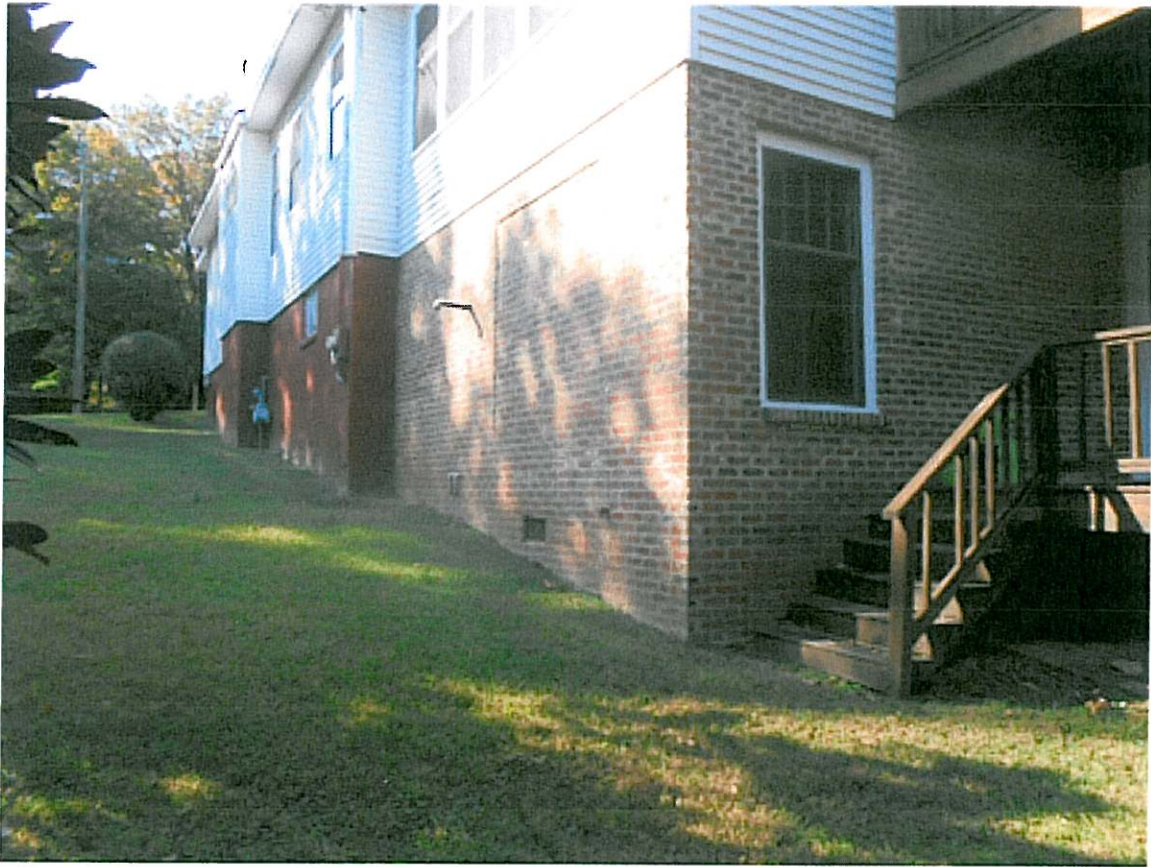
FOUNDATION WALL ON SLOPING LOT
