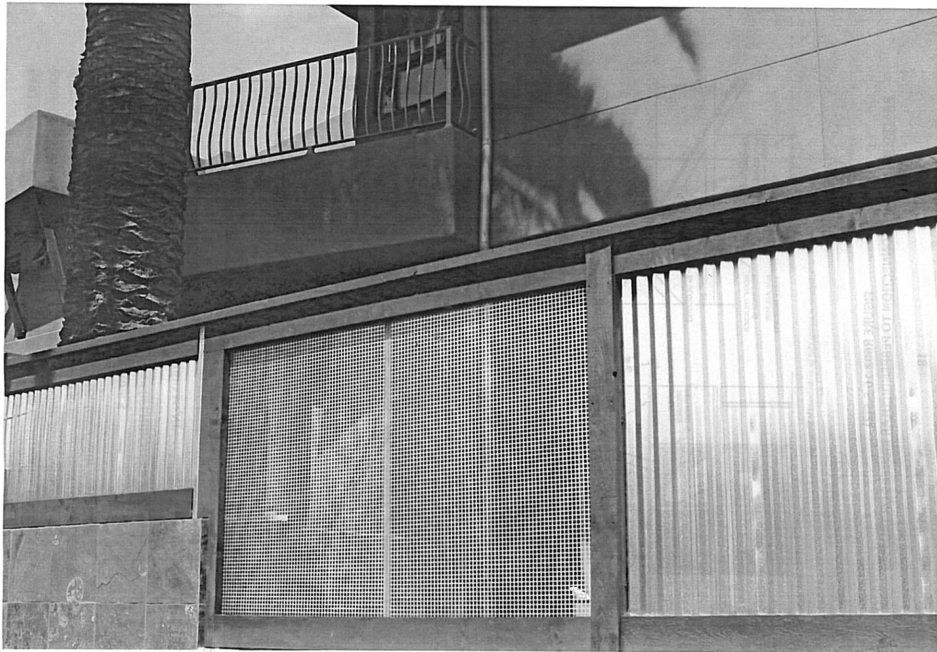
WOOD FRAMED FENCING DETAIL (CORRUGATED METAL PANEL INSERTS)
