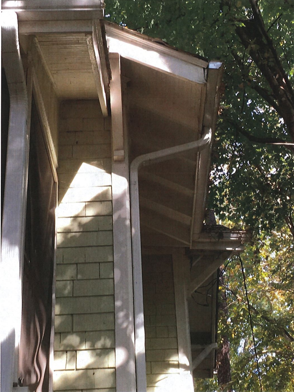
Photo 5: Existing roof overhang and brackets
