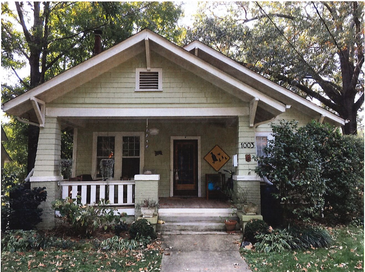
Photo 1: View from street (North elevation)
