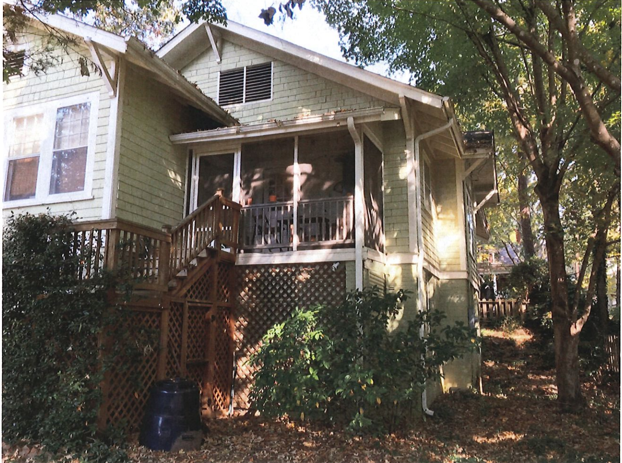
Photo 3: Existing screened in porch at back of house
