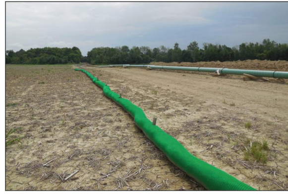
Filtrexx SiltSoxx ORIGINAL used as Perimeter Control.
