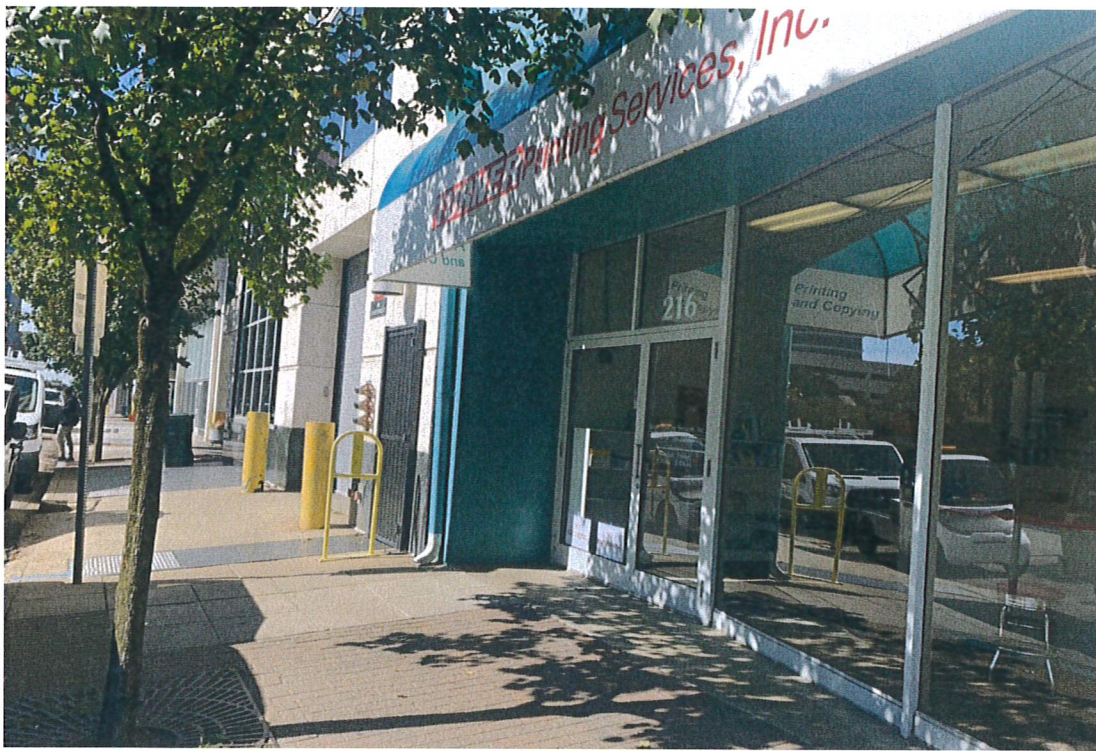
Close-up view of non-original storefront
