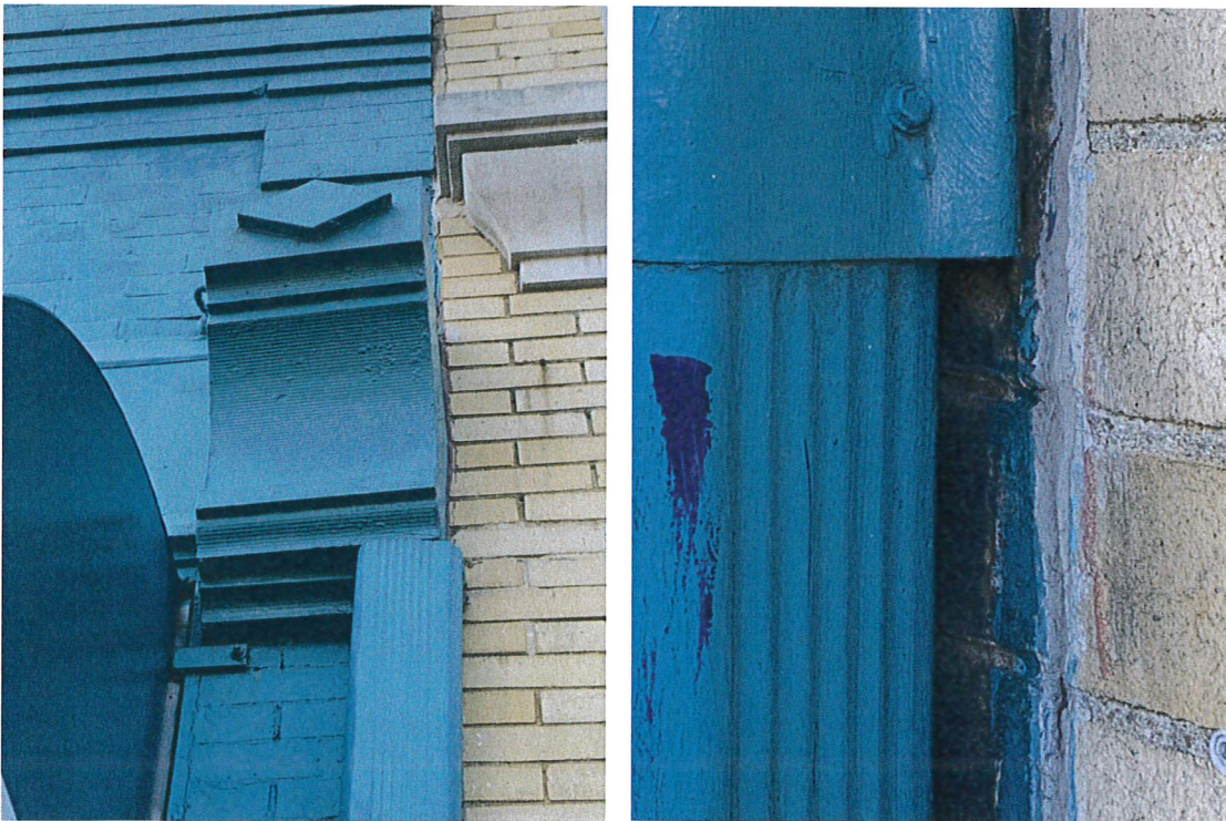
Close-up view of metal conductor head and roof leader (L) and unpainted brick (R)
