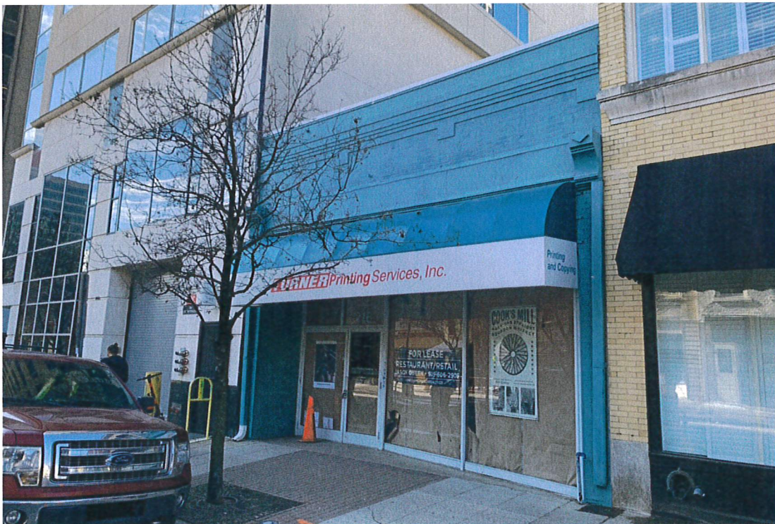
View of façade from northeast
