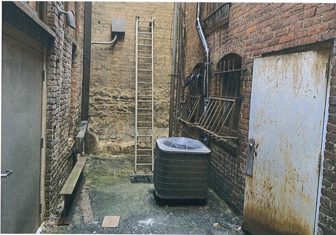
View of roof rear courtyard looking north. Subject building is on the right. Proposed changes are limited to: 1) replacing the existing rear hollow metal door with a full lite hollow metal door, 2) reglazing the existing steel window frames if/as needed, and 3) adding a wall-mounted condenser at the top floor.
