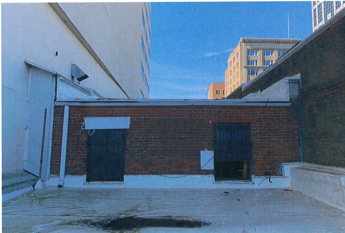
View of roof looking west. There are no proposed changes to this façade with the exception of reglazing the existing windows.
