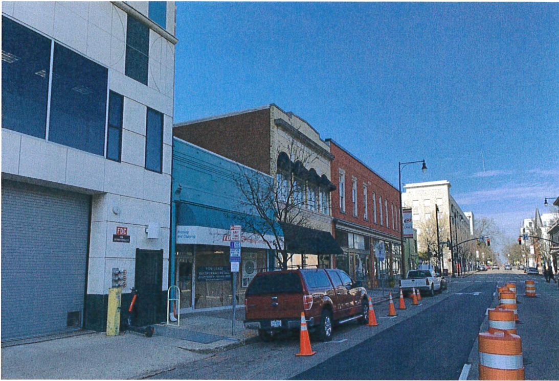
Context view looking north on Wilmington Street
