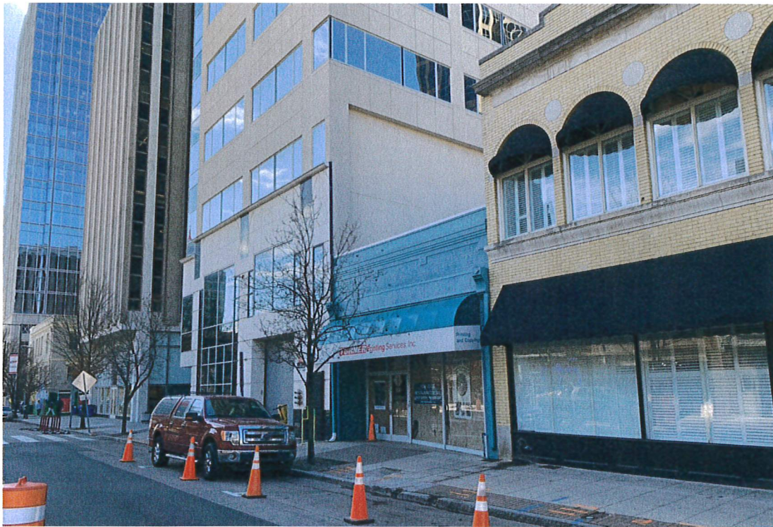
Context view looking south on Wilmington Street
