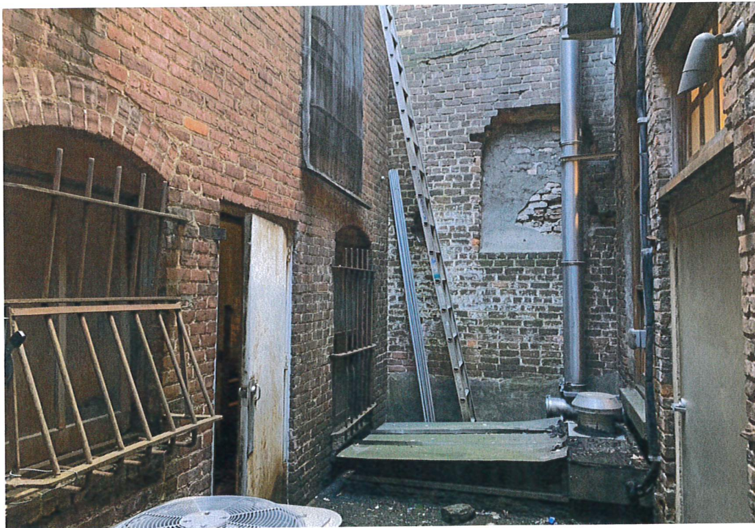
View of roof rear courtyard looking south. Subject building is on the left. Proposed changes are limited to: 1) replacing the existing rear hollow metal door with a full lite hollow metal door, 2) reglazing the existing steel window frames if/as needed, and 3) adding a wall-mounted condenser at the top floor.
