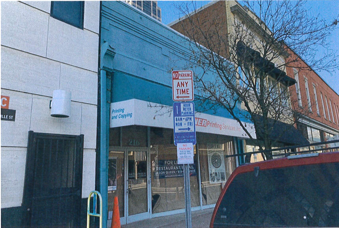
View of façade from southeast
