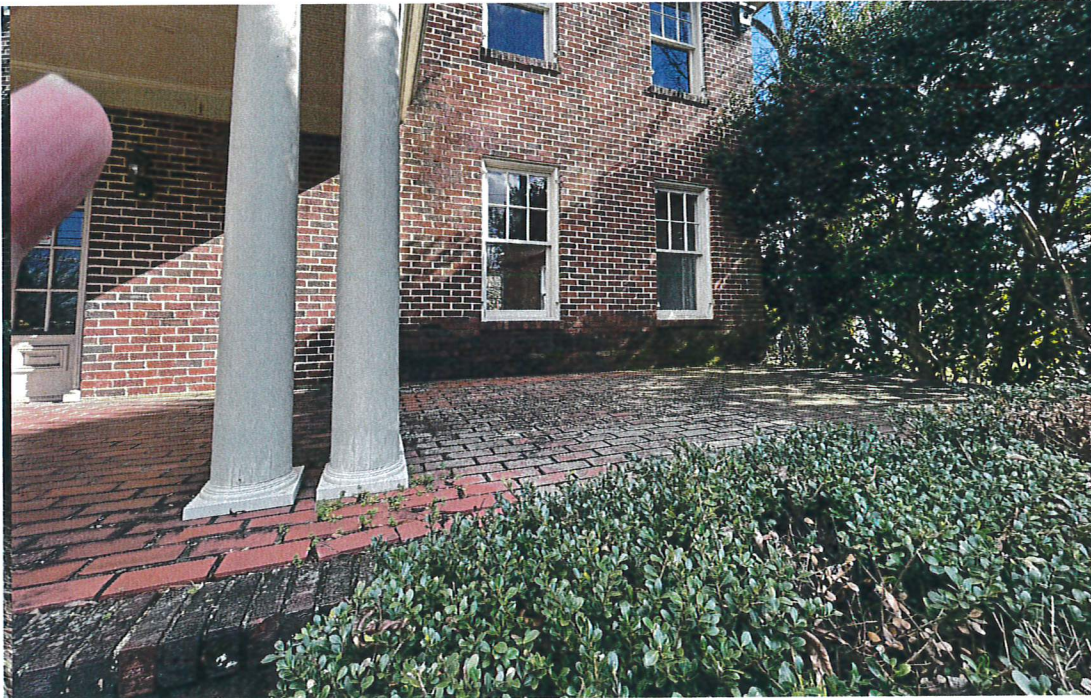
1 FRONT PORCH FLOORING TO BE REPLACED Scale: N/A
