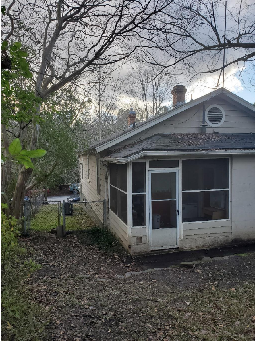
Photograph #4: South/ East Elevation w/ Addition to Be Removed
