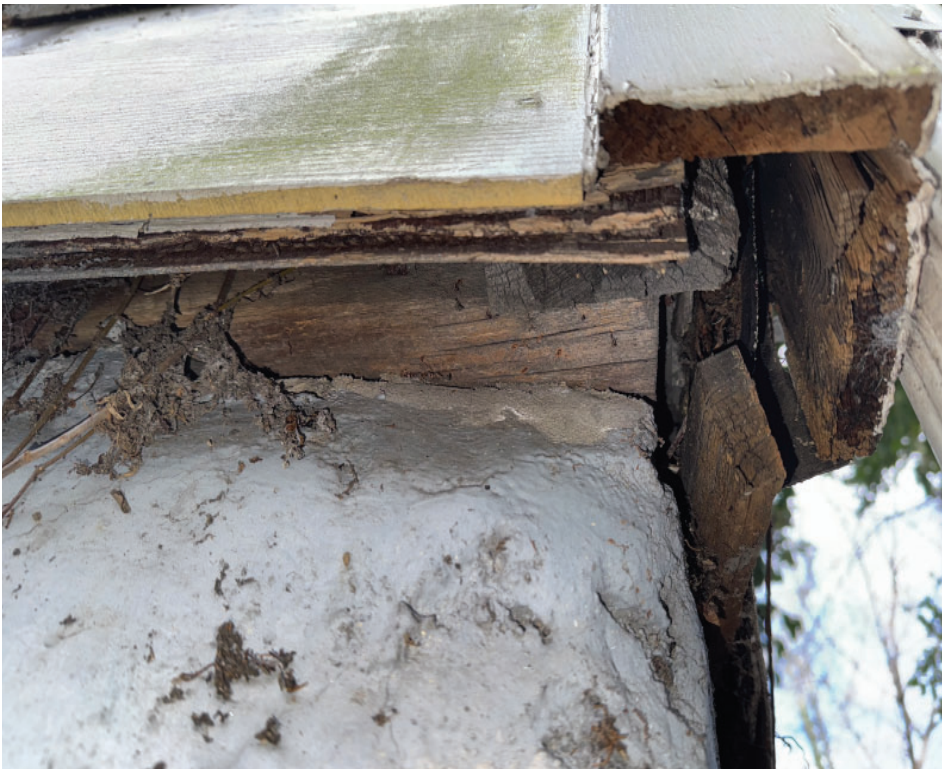
36 - EXTERIOR VIEW OF LAYERS OF SIDING AND TRIM OVER FOUNDATION CORNER
