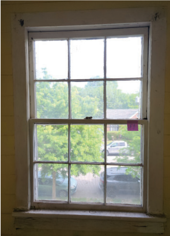
31 - F1 WINDOW INTERIOR VIEW- TYPICAL UPPER LEVEL WINDOW- NO ROPE SASHES
