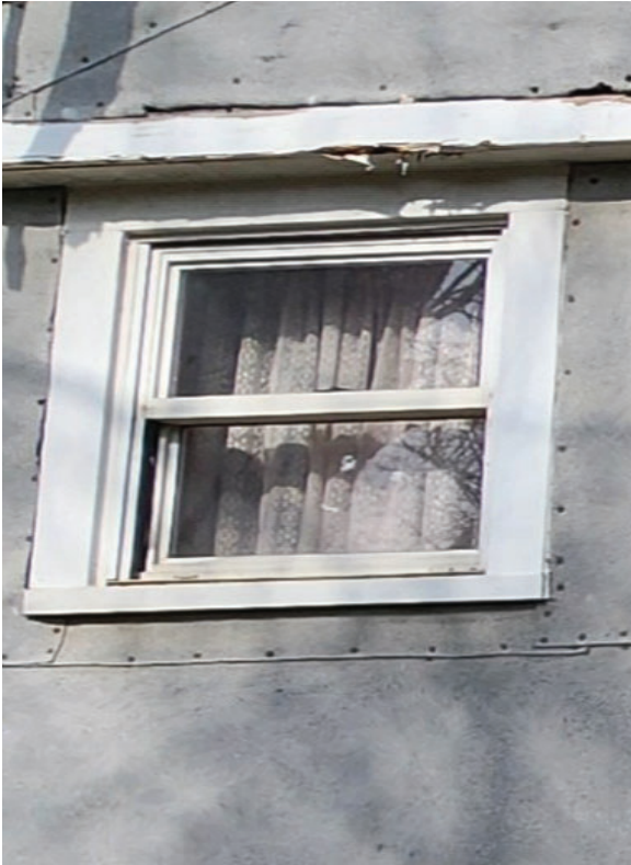
33 - C1 WINDOW EXTERIOR DETAIL- NON ORIGINAL VINYL WINDOW
