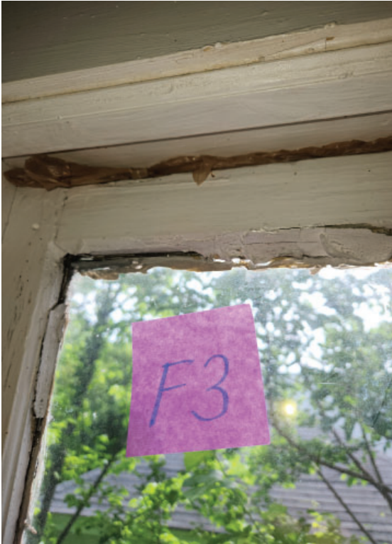
35 - F3 WINDOW-TYPICAL DETERIORATION
