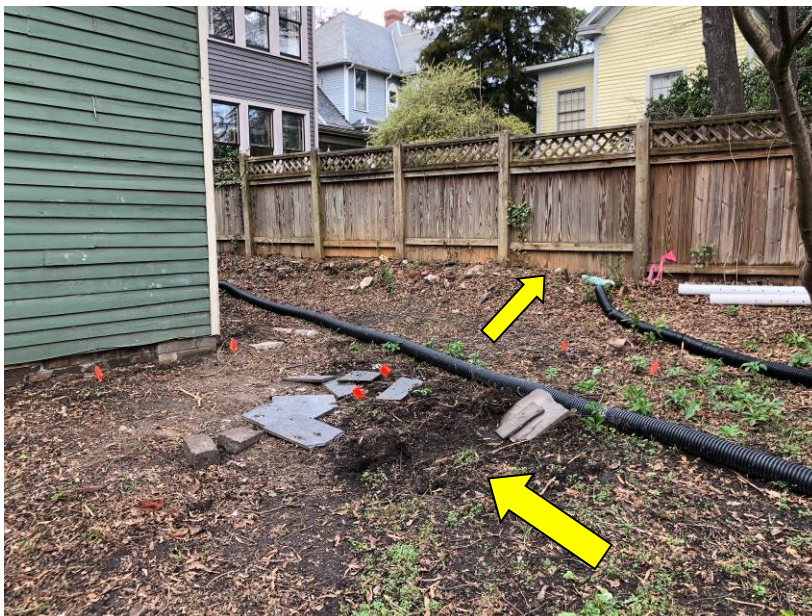
Photo: standing in back yard looking north west towards the house. Note slate foot path that had been buried by runoff (unearthed by the Morgans and proposed for re-use in new patio). Also note green PVC drainage pipe under fence that will need to be relocated as part of the water management proposal.
