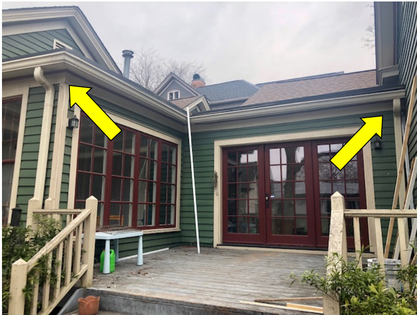
Photo: existing square gutters and downspouts on south side of home.
