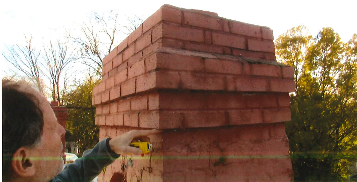
02 - Chimney 3 with rebuilt cap
