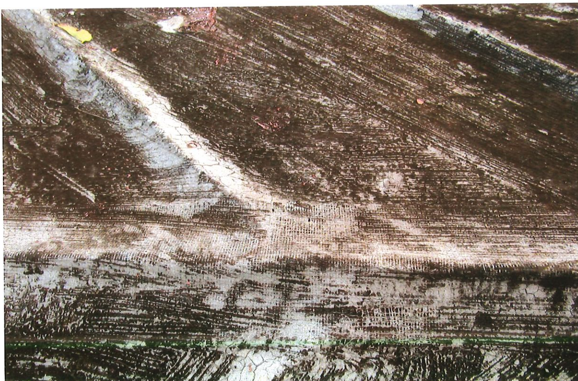
14 - Existing roof covered in fiberglass and tar
