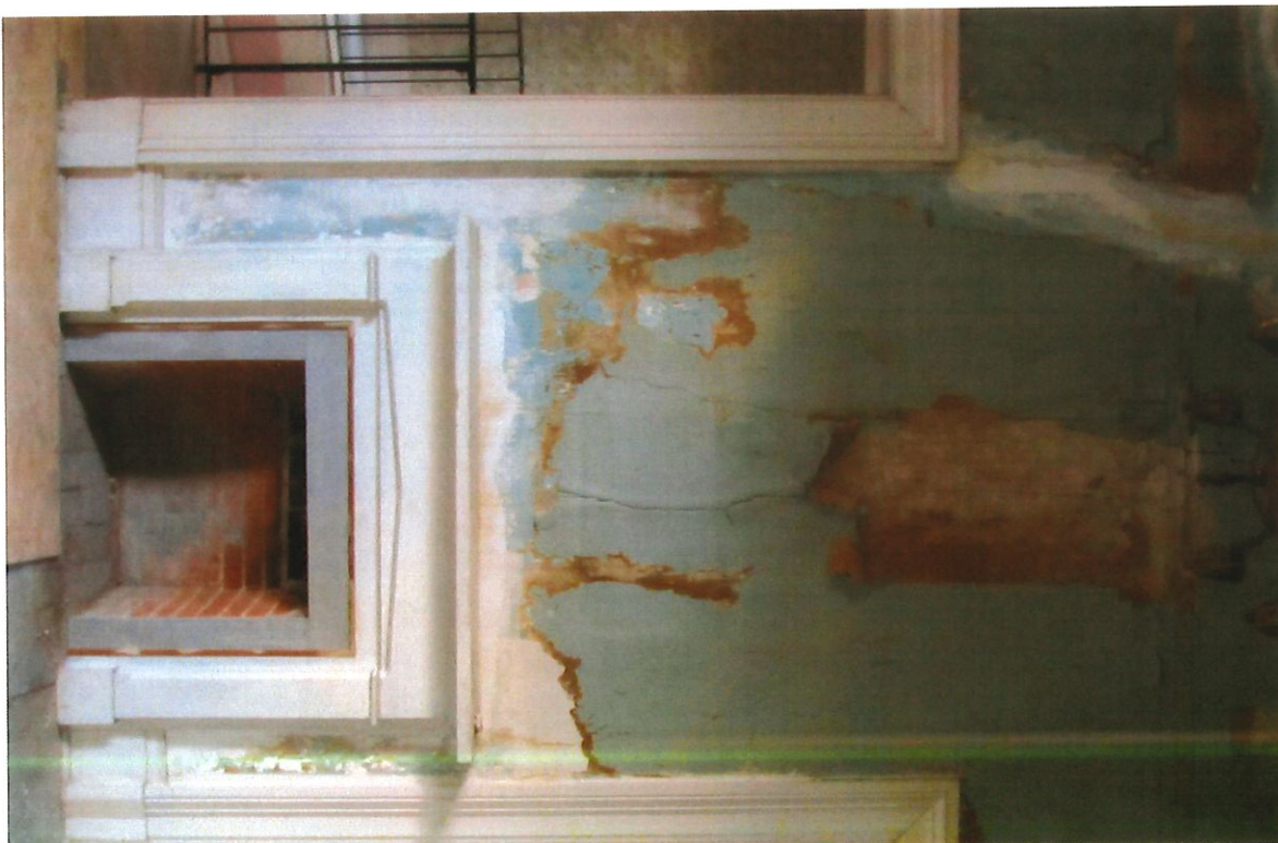
16 - Second floor bedroom below chimney 2 - note water damage above mantle
