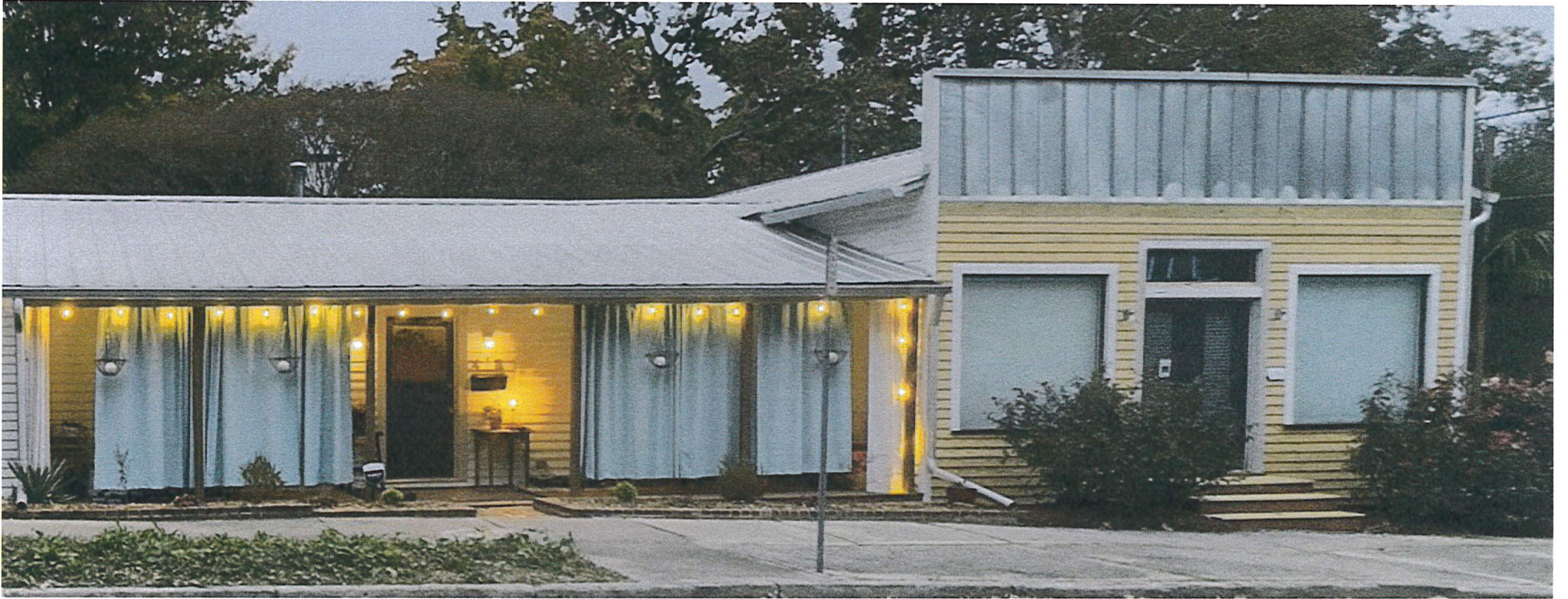
415 N. Boundary St. East side of property
