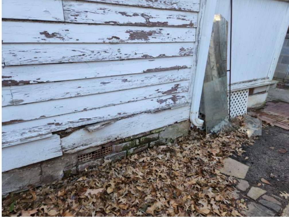
EXAMPLE OF ROTTEN DRIP CAP/SIDING TO BE REPLACED IN KIND
