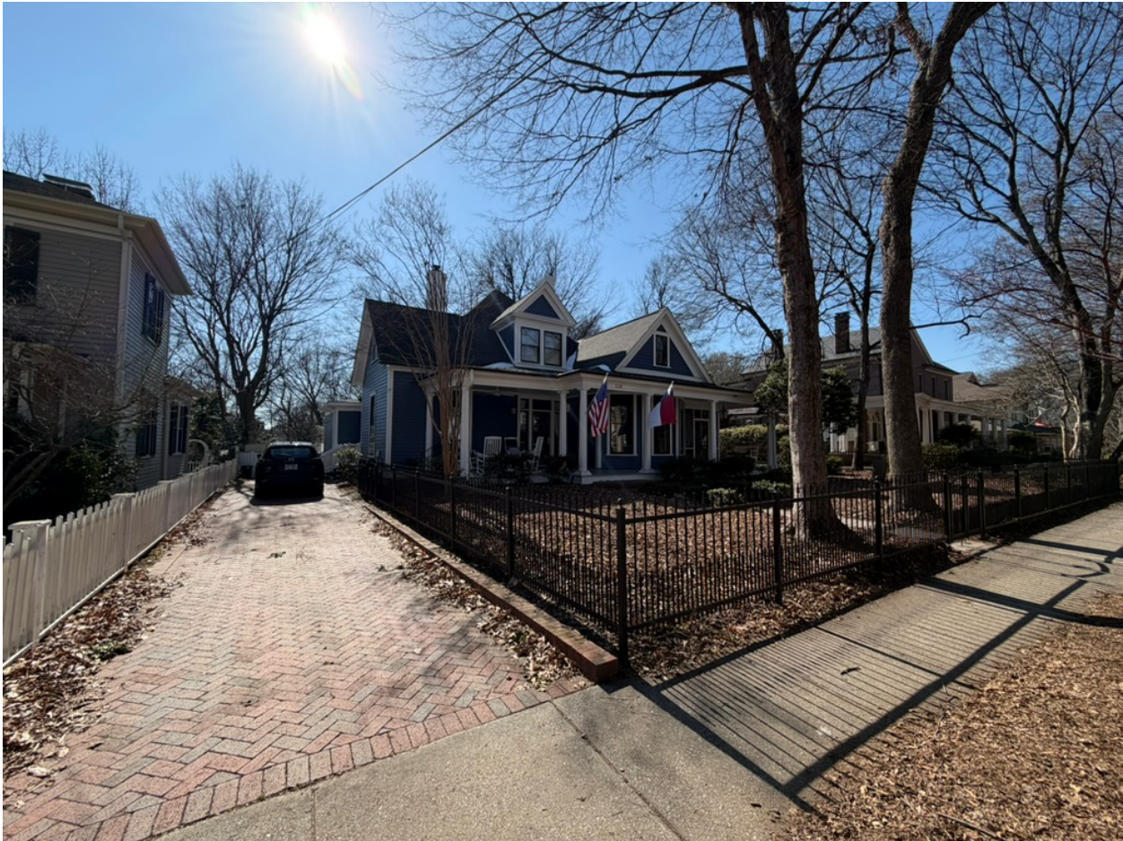
North-east corner, facing west (528 E Jones)
