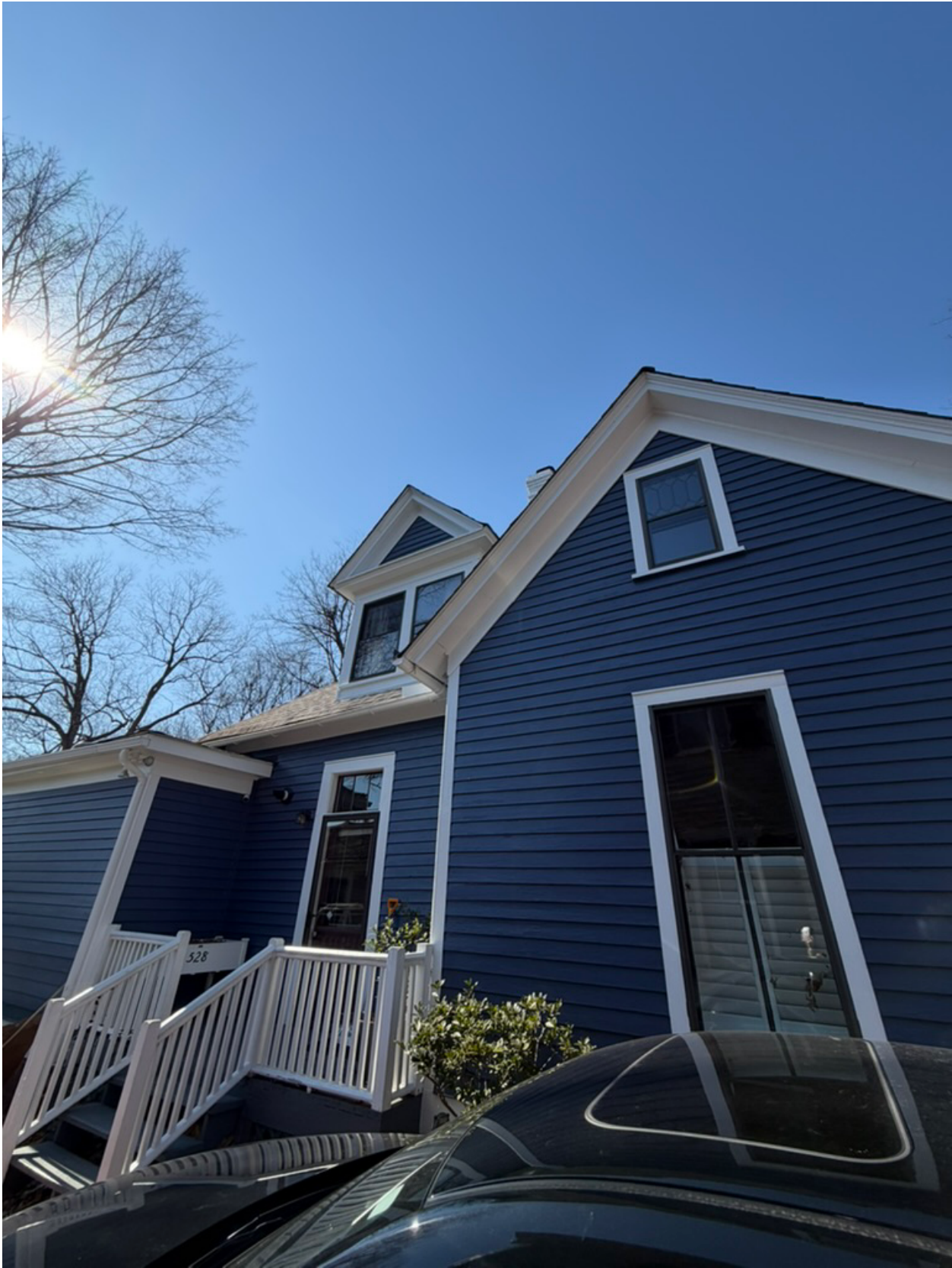
East-facing side of the house (528 E Jones)
