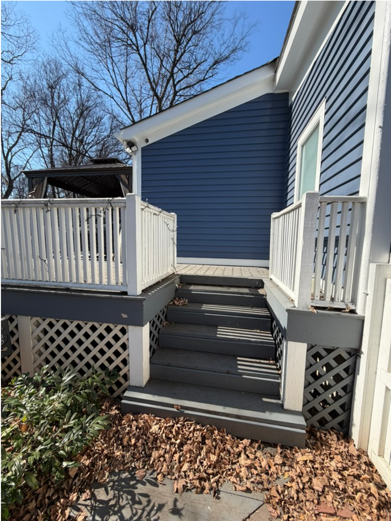
East-facing side of the deck. We plan to remove these stairs.
