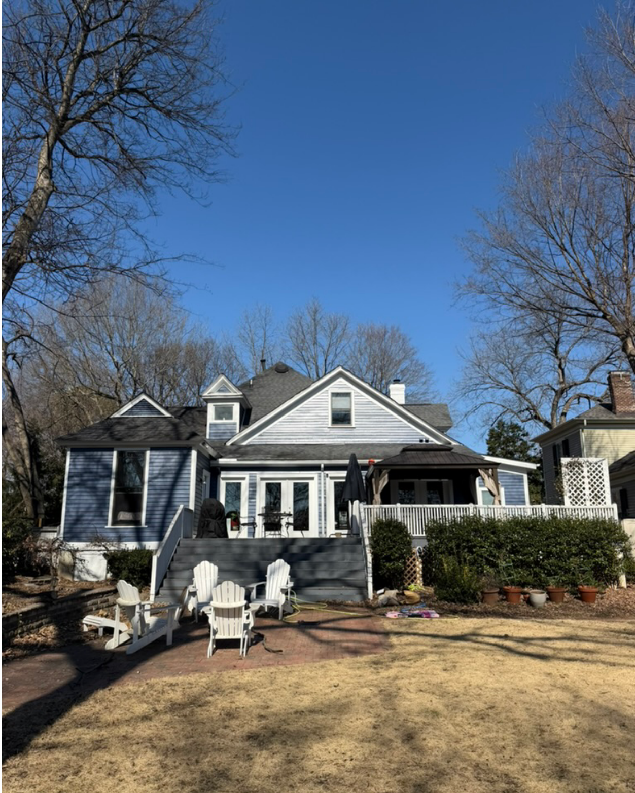
South-facing side of the house. Current deck has exceptionally wide stairs, which we'd like to narrow. The structure on the right is a temporary screened porch the previous owners installed — we plan to remove it. The sauna will be located on the deck, on right side (east side). (528 E Jones)
