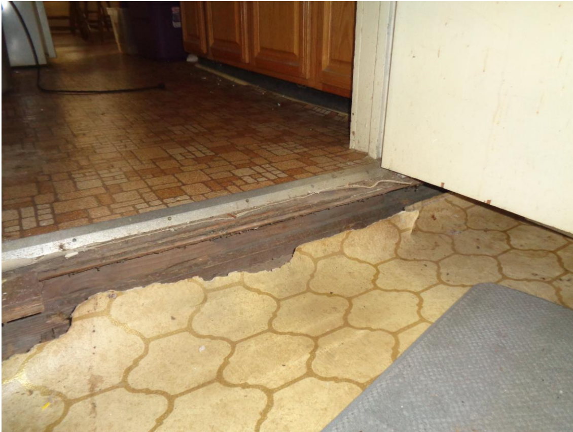
Photo 12A: Existing sunken floor at existing kitchen
