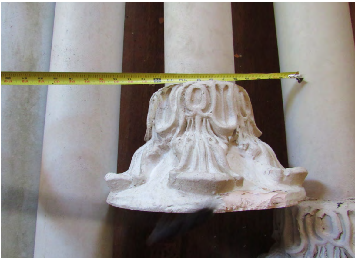
14 - 'Temple of the Wind' column capital cast around PVC column
