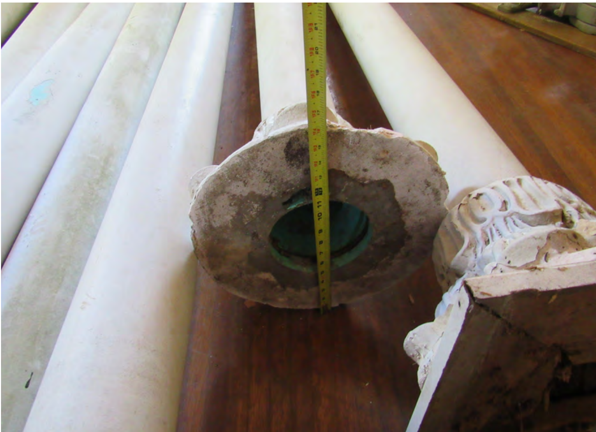
12 - 'Temple of the Wind' column capital cast around PVC column
