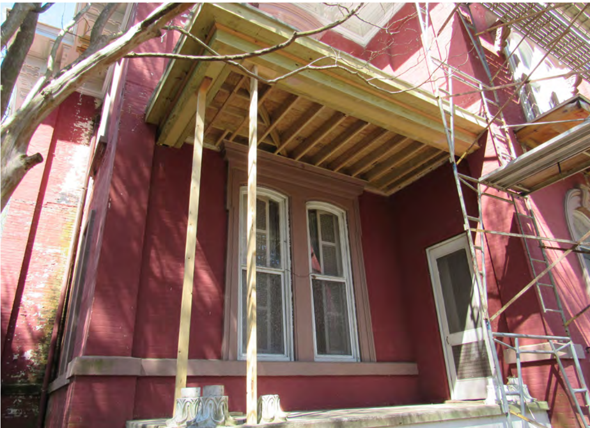
08 - South porch with roof repair in process. Several column bases remain attached to concrete slab
