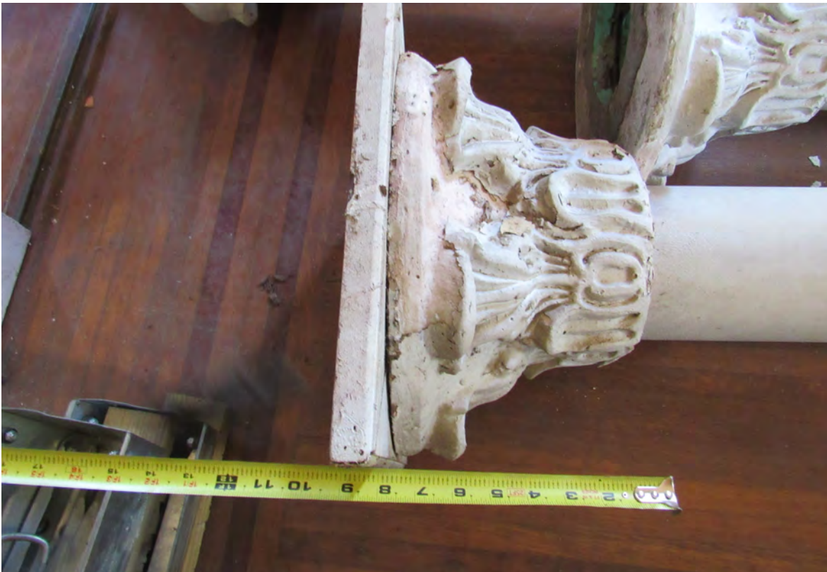
13- 'Temple of the Wind' column capital cast around PVC column
