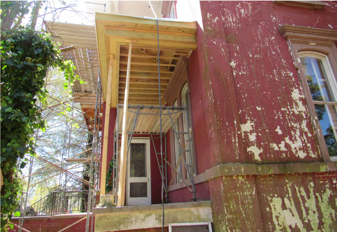
09- North porch during roof repair. Column base still attached to concrete slab at porch floor
