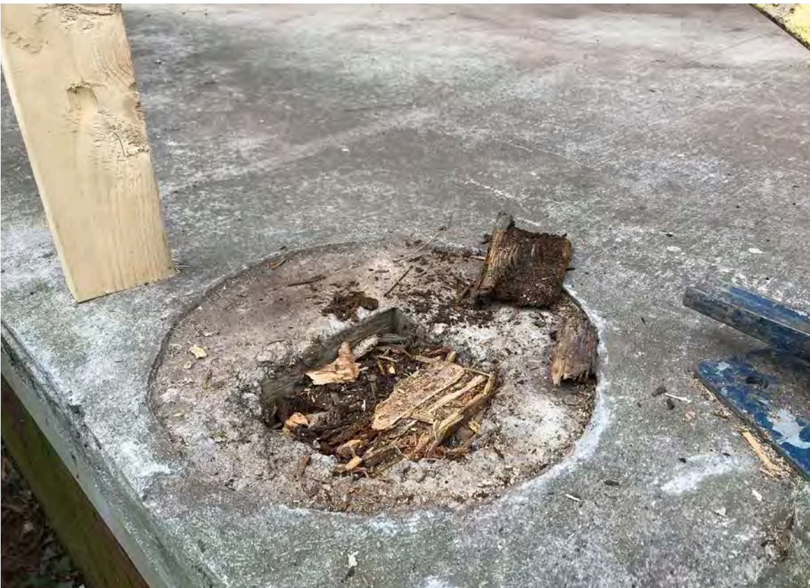
10 - North porch concrete slab showing cast in place base around 6x6 wood post
