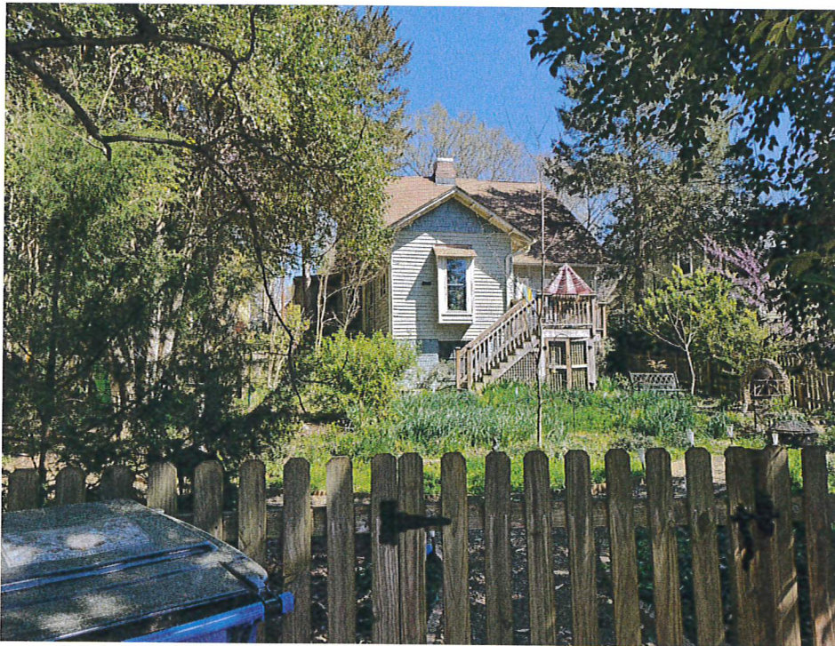
Back view from alley
