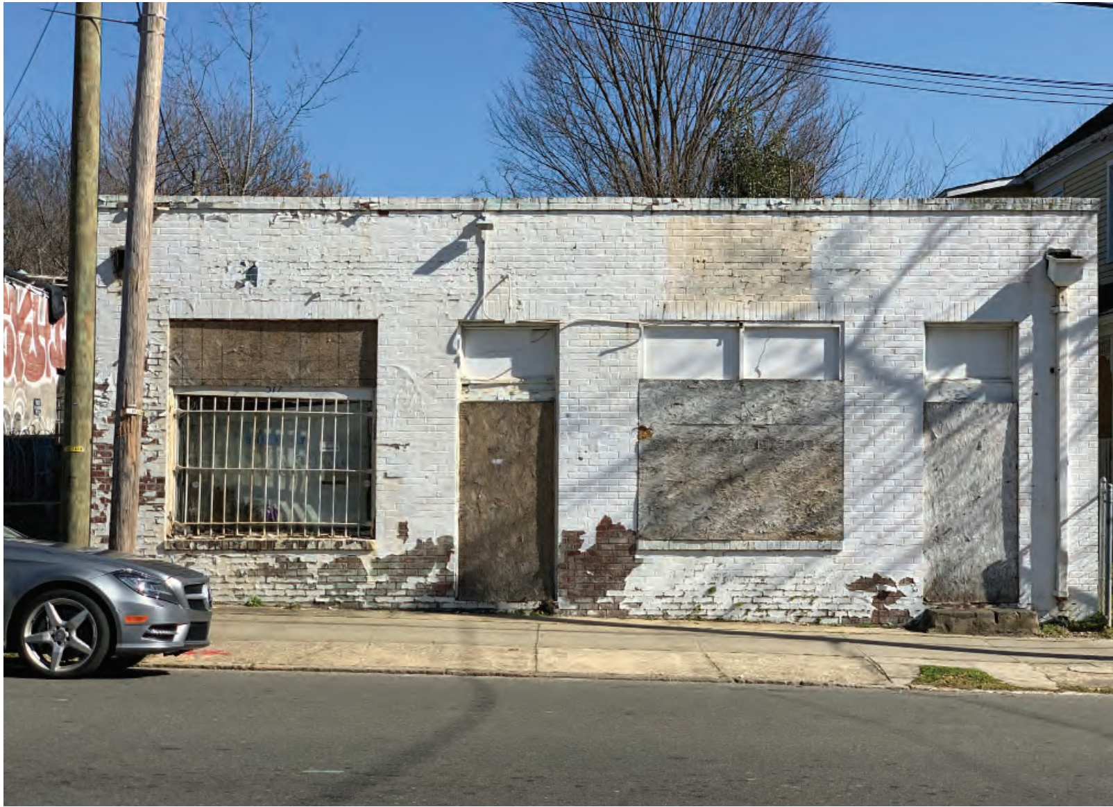
WEST FACADE - RESTORE PAINTED WOOD STOREFRONT AND DOORS. SALVAGE GLASS AND CHECK CASHING SIGNAGE ON LEFT WINDOW, PROVIDE ADA ENTRY RAMP UP TO LEFT ENTRY DOOR.
