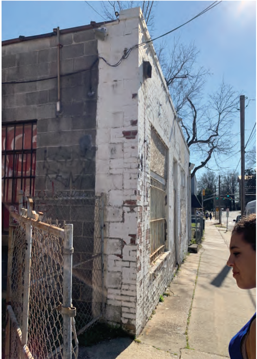
STREET + NORTH FACADE - RESTORE BRICK DETAILING, REMOVE PAINT FROM CMU - REMOVE PAINT FROM BIRCK , REPOINT AS NEEDED,
