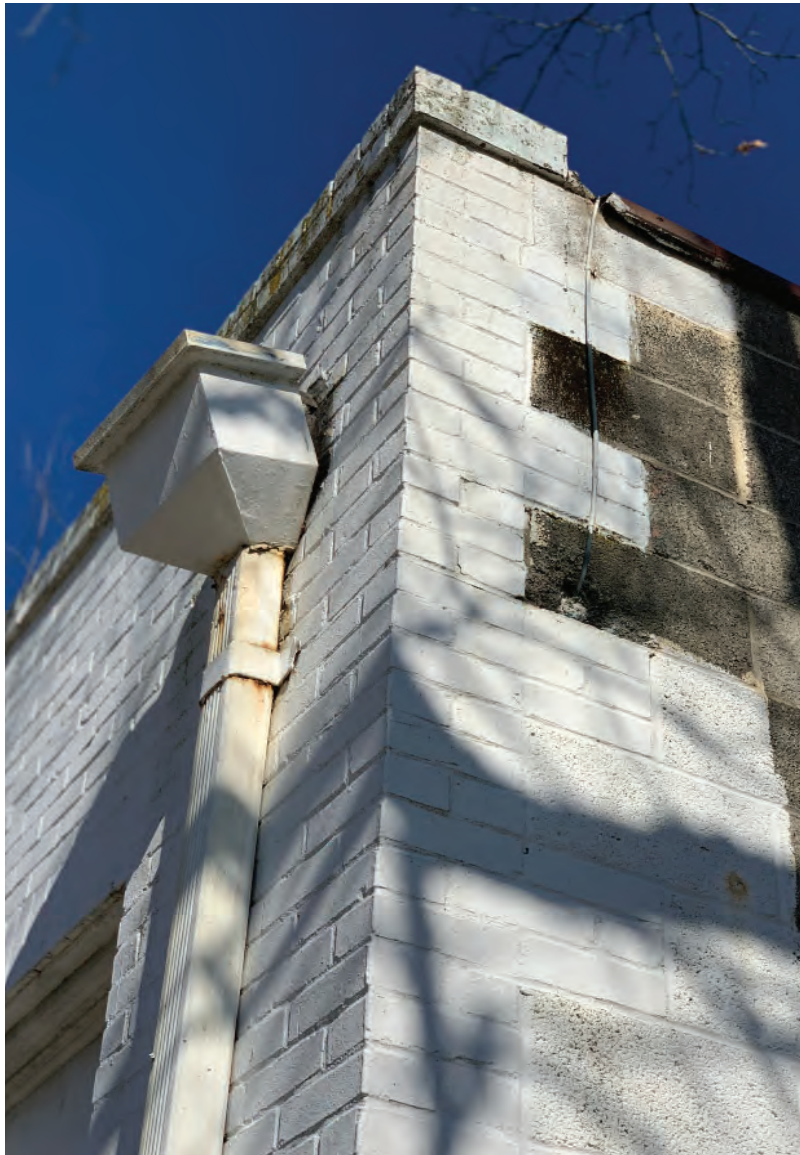
WEST + SOUTH FACADE - RESTORE BRICK DETAILING, REMOVE PAINT, REPLACE EXISTING DOWNSPOUT
