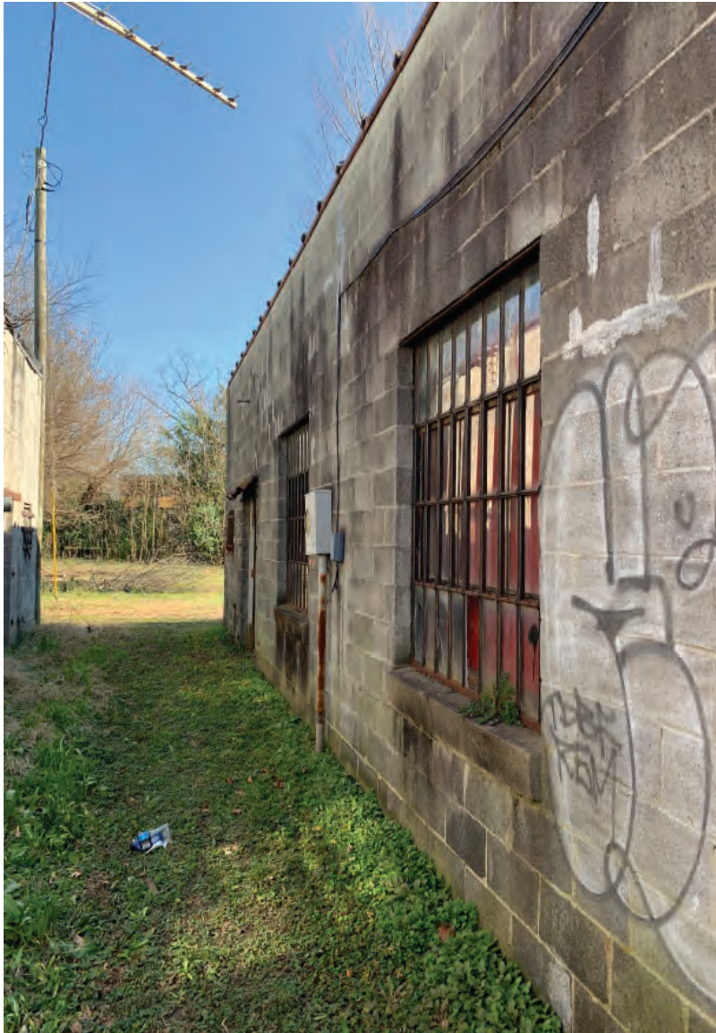
NORTH FACADE - EXISTING WINDOWS - REPLACE GLASS WHERE NEEDED, REAPPLY TERRACOTTA COPING
