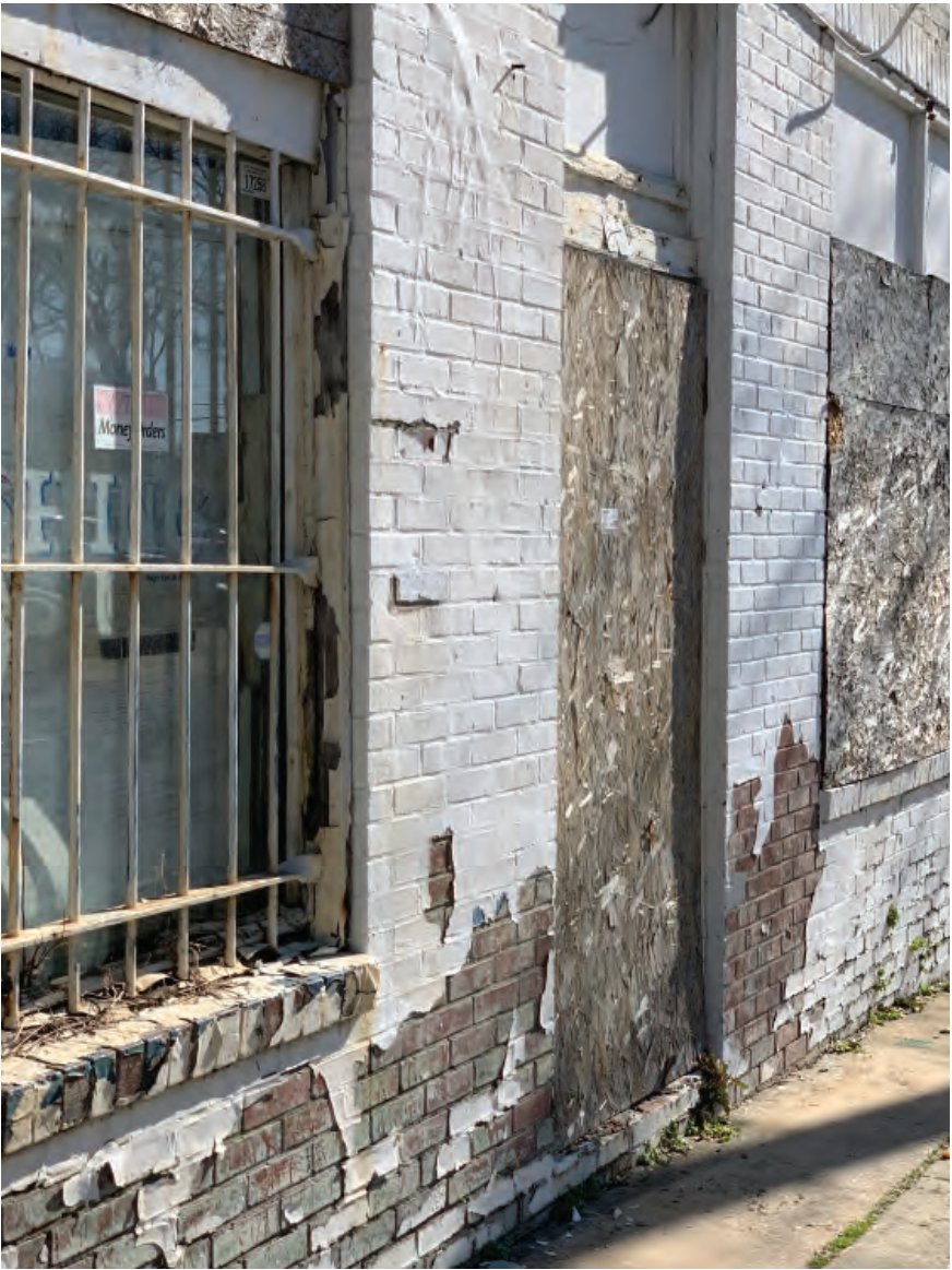
WEST FACADE - REMOVE WINDOW BARS, RESTORE EXISTING WOOD STOREFRONT WINDOWS AND DOORS
