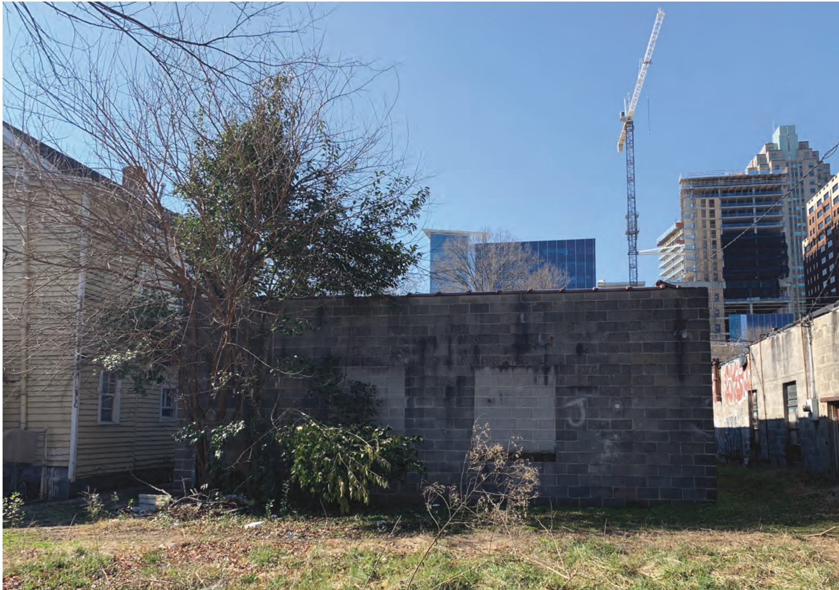
NEW OPENING WHERE EXISTING PUNCHED WINDOWS WERE INFILLED
