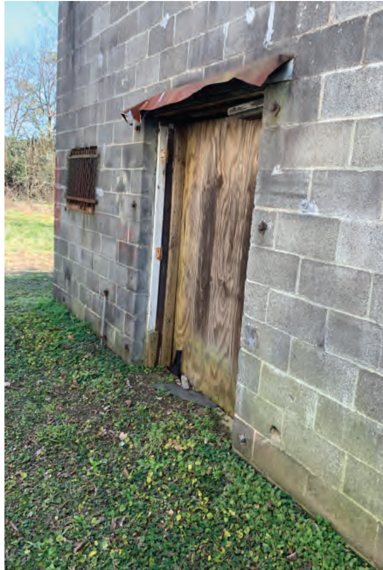
NORTH FACADE- REPLACE DOOR WITH WINDOW, REMOVE BARS FROM WINDOW REMOVE METAL OVERHANG,
