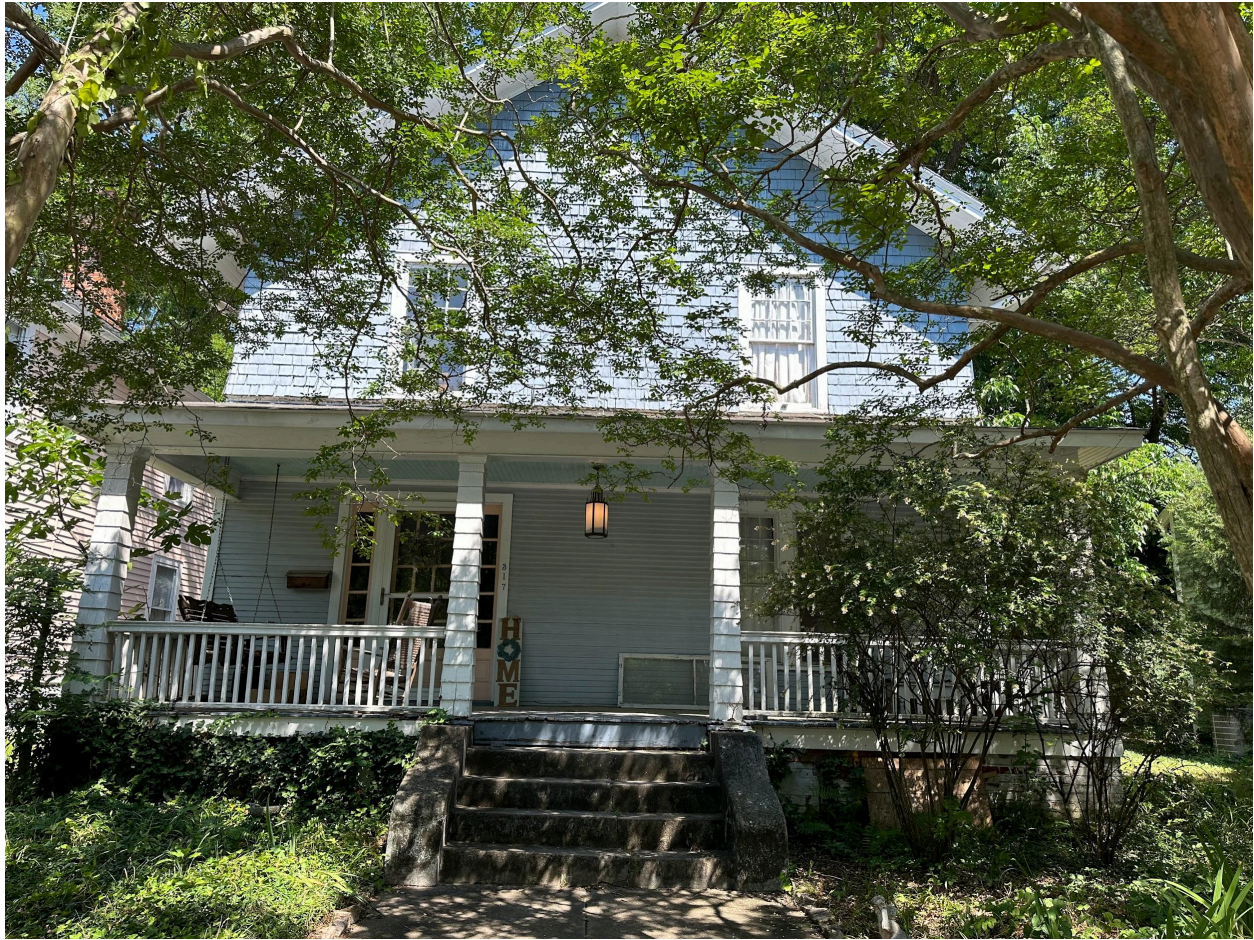
Front - West Facing
