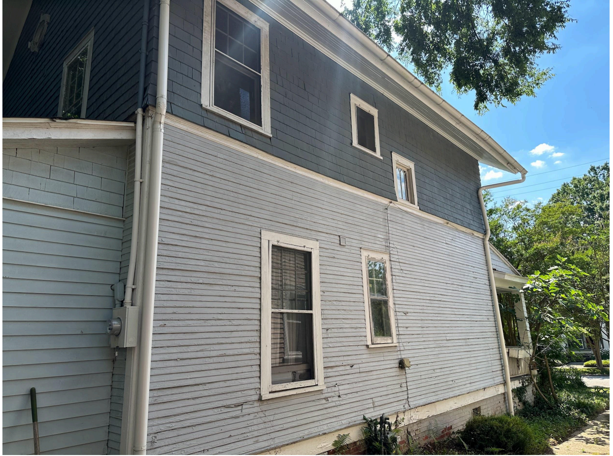
Side - North Facing
