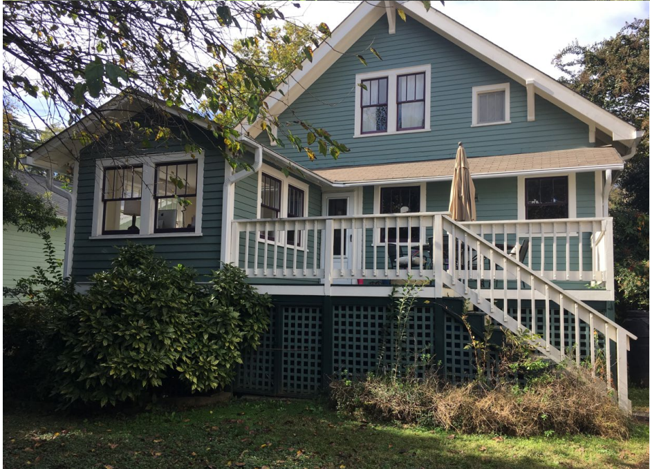
Rear Exterior View
