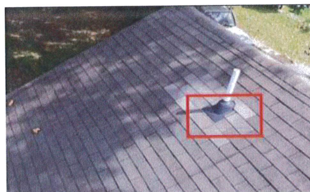
3.1 Item 1(Picture) Plumbing boots not completely secured
