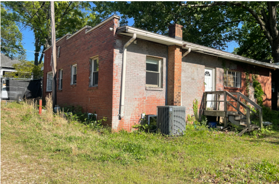
04 - Existing northwest corner of building
