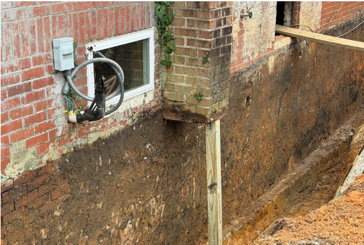
01 - View of bottom of chimney during waterproofing (most recent)
