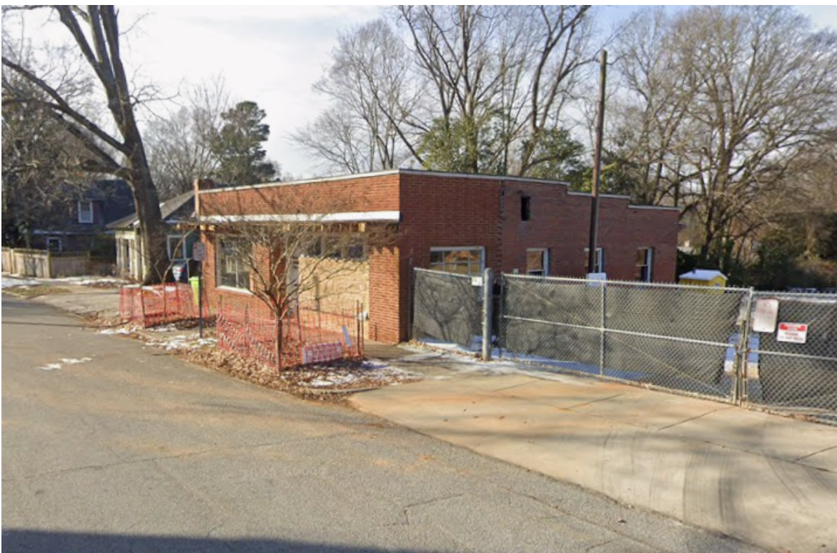
02 - Existing northeast corner of building
