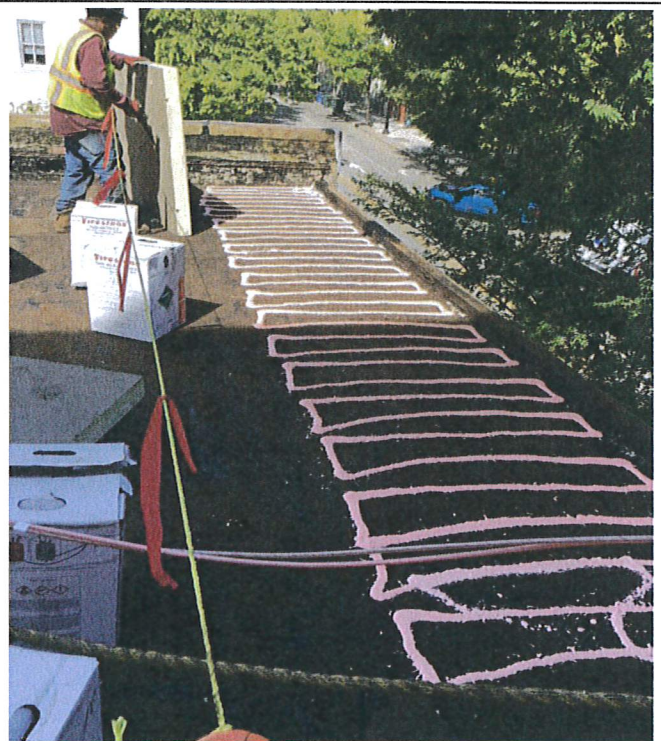
Adhered insulation being installed
