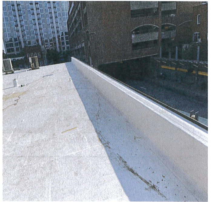
Wall Flashing
