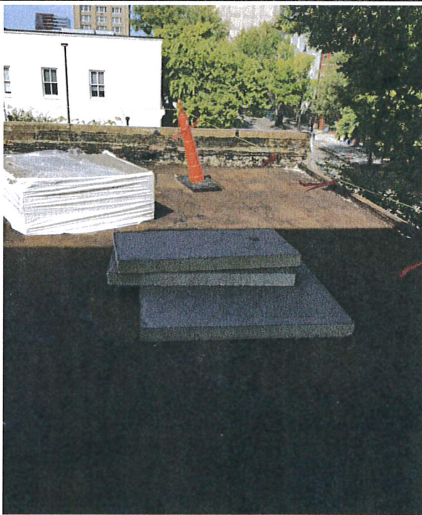
Built- up removed roof cleaned
