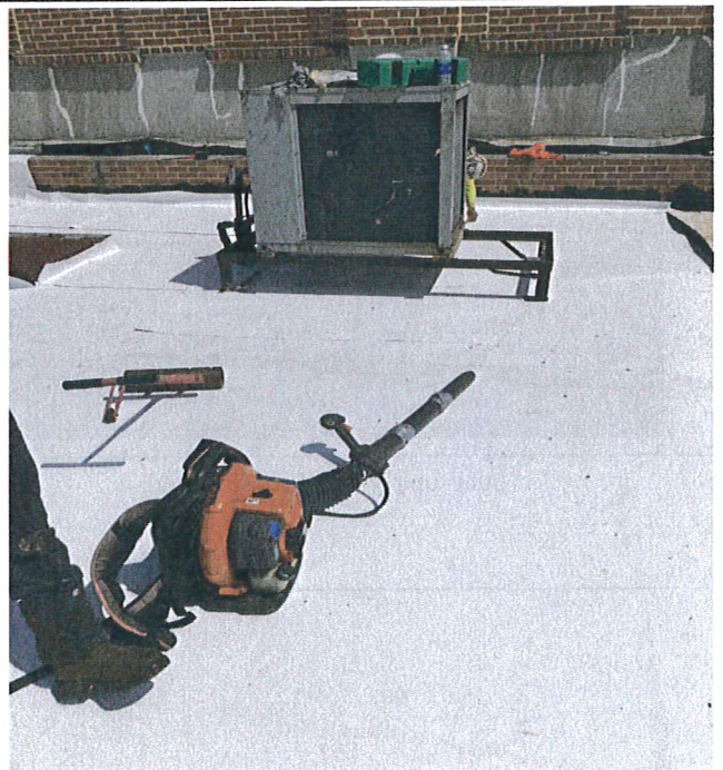
60Mil self-adhered membrane
