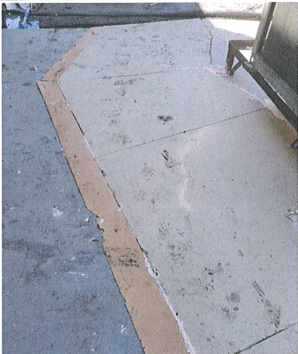
Progress work/ 4" insulation adhered to concrete deck
