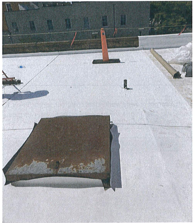
60Mil self-adhered membrane
