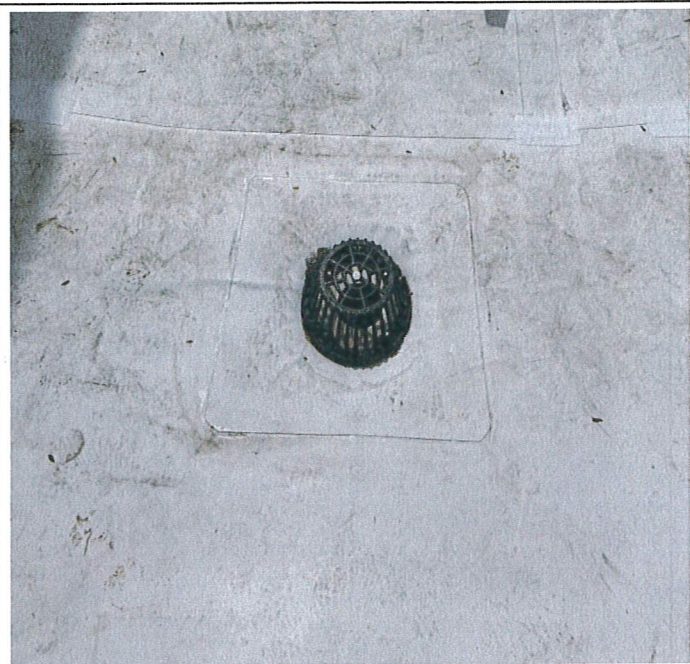
New Drain installed
