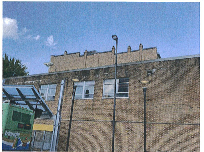
Gravel Stop Metal (Ground View)
