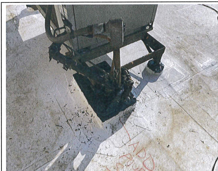
Pitch Pockets/ corner flashing
