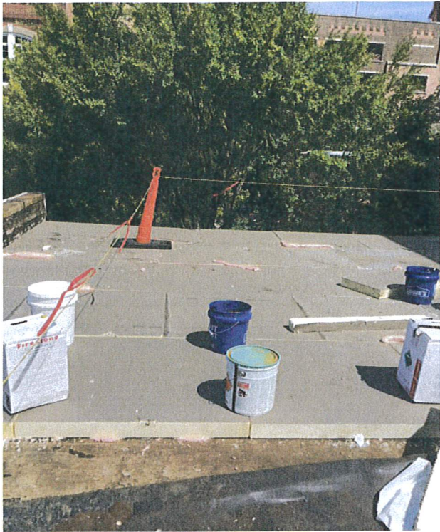
Progress work/ 4" insulation adhered to concrete deck
