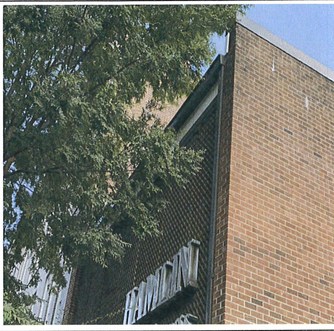
Gutter Down Spout
