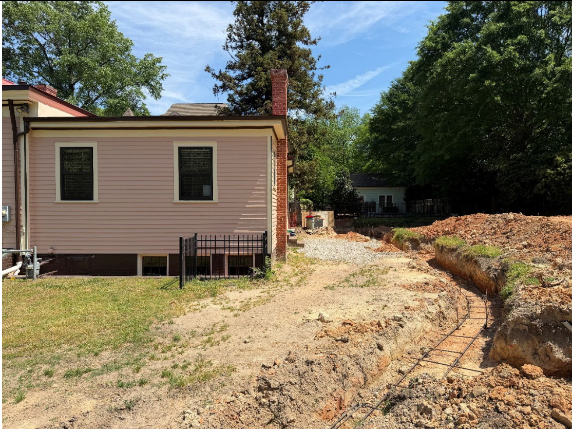
West Side of House and Property (View from North East Street)
