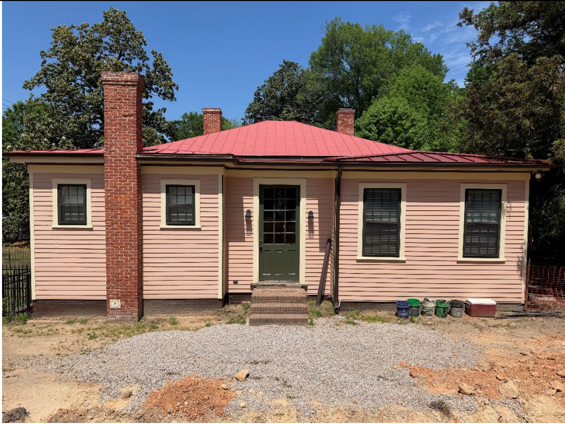
Rear of House (South Side)
