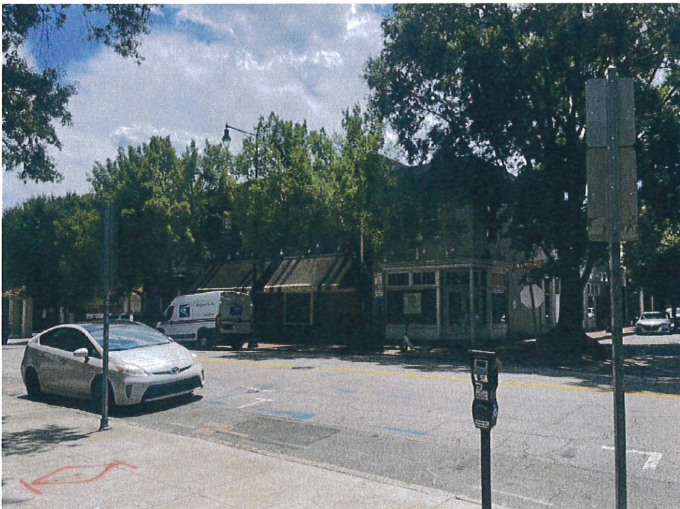
02 - Existing north or main elevation from across Martin st.
