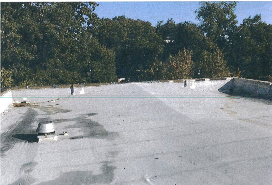
10 - View of existing roof
