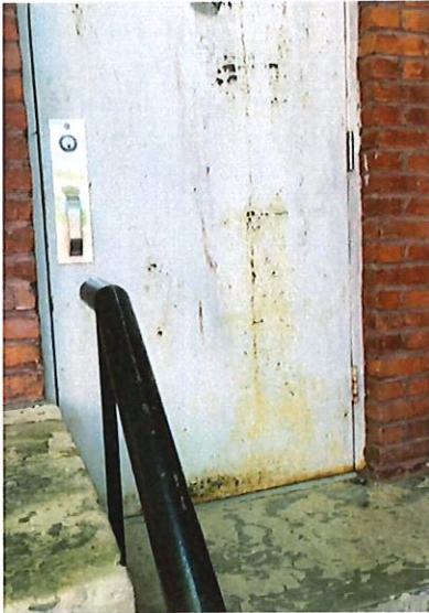
Existing exterior hollow metal doors and frames (not original bldg. features)
