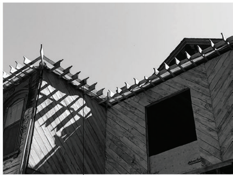
NEW CEILING JOIST/SOFFIT FRAMING UNDER CONSTRUCTION AT REAR UPPER ADDITION, TYP. AT ALL EPDM ROOFS
